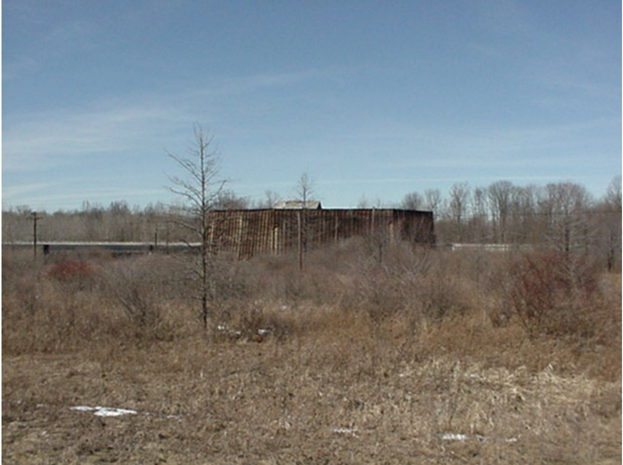
Figure 2-1. Site Conditions at Load Line 4, March 2003
