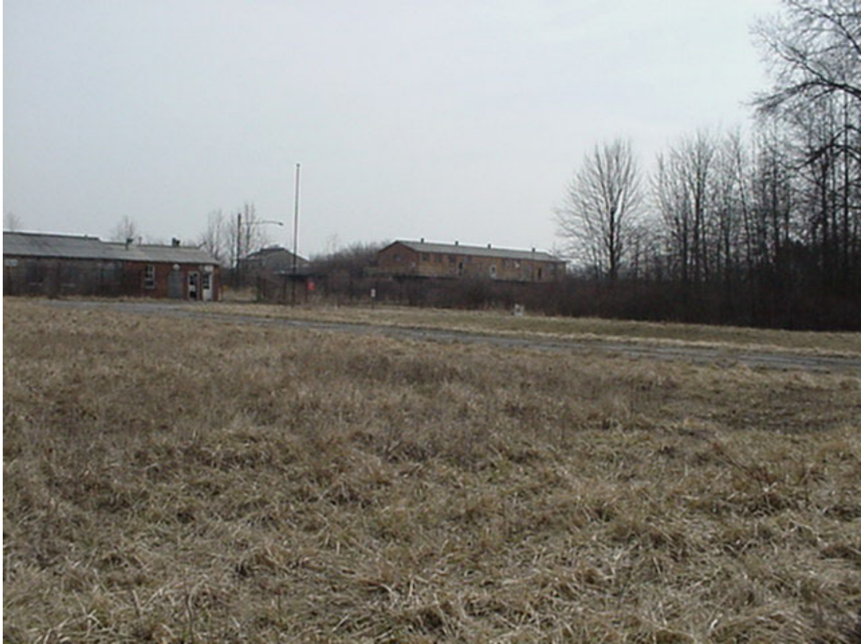
Figure 2-1. Site Conditions at Load Line 3, March 2003
