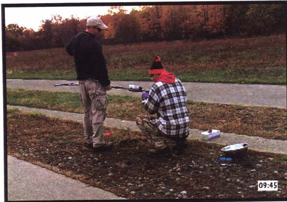
SAIC Using Hand Auger After UXO Clearance
