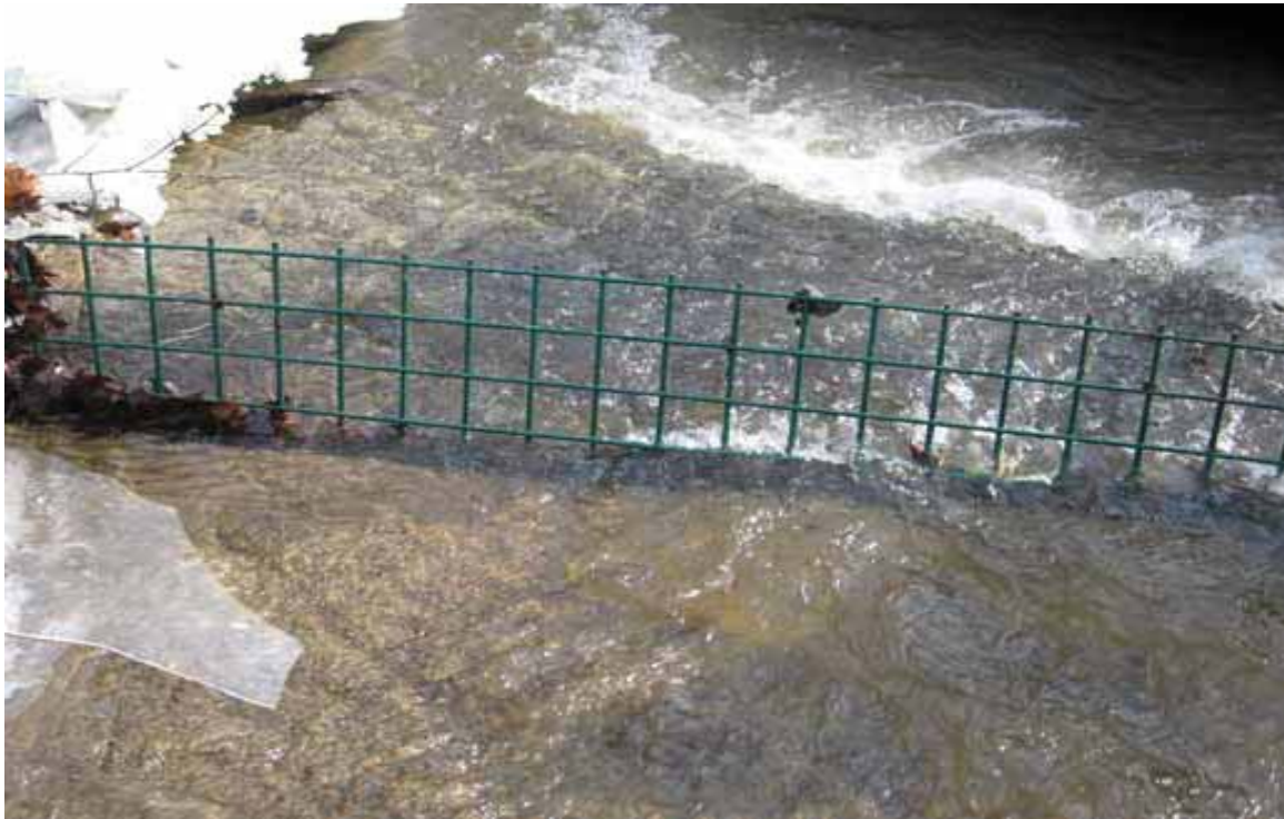
CLOSEUP OF UPSTREAM BARRIER FOLLOWING CLEANUP.
