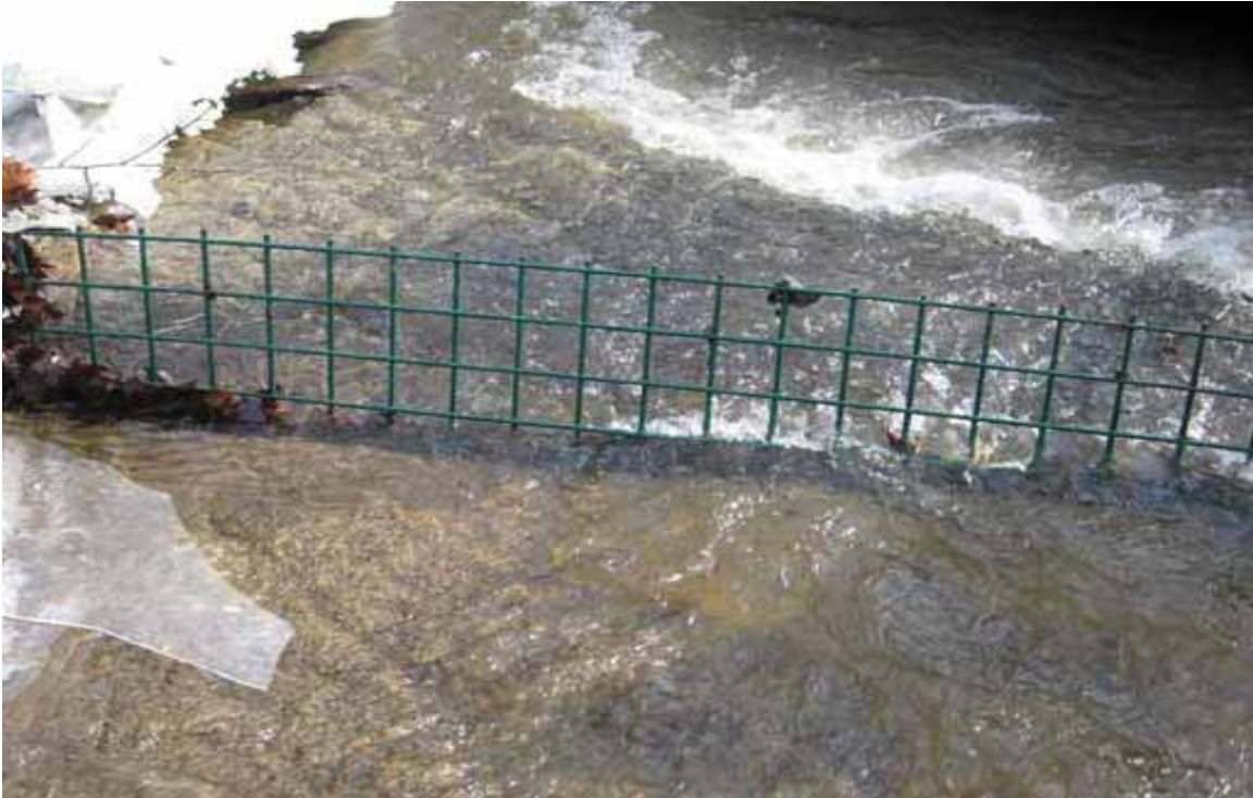
CLOSEUP OF UPSTREAM BARRIER FOLLOWING CLEANUP.
