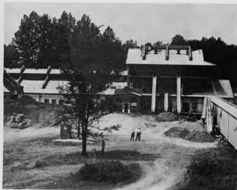
Workers built a protective earth barricade along one of the production lines.
