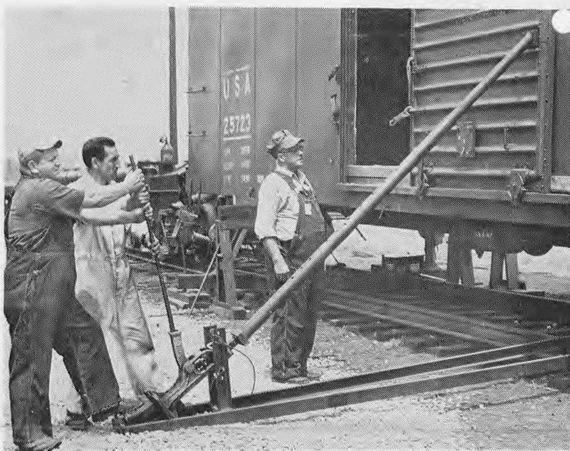
A $200 SUGGESTION award was presented to J. C. Shanks, Railroad Shop Maintenance, for his "jig" to straighten buckled, steel doors on Arsenal freight cars. Mr. Shanks (left), and John Urban are shown using the "jig" to straighten a car door. Watching the operation is Homer Zimmerman, department foreman. The "jig" will also straighten buckled sides of box cars without the application of heat. Mr. Shanks is a Newton Falls resident and a first-time idea winner.
