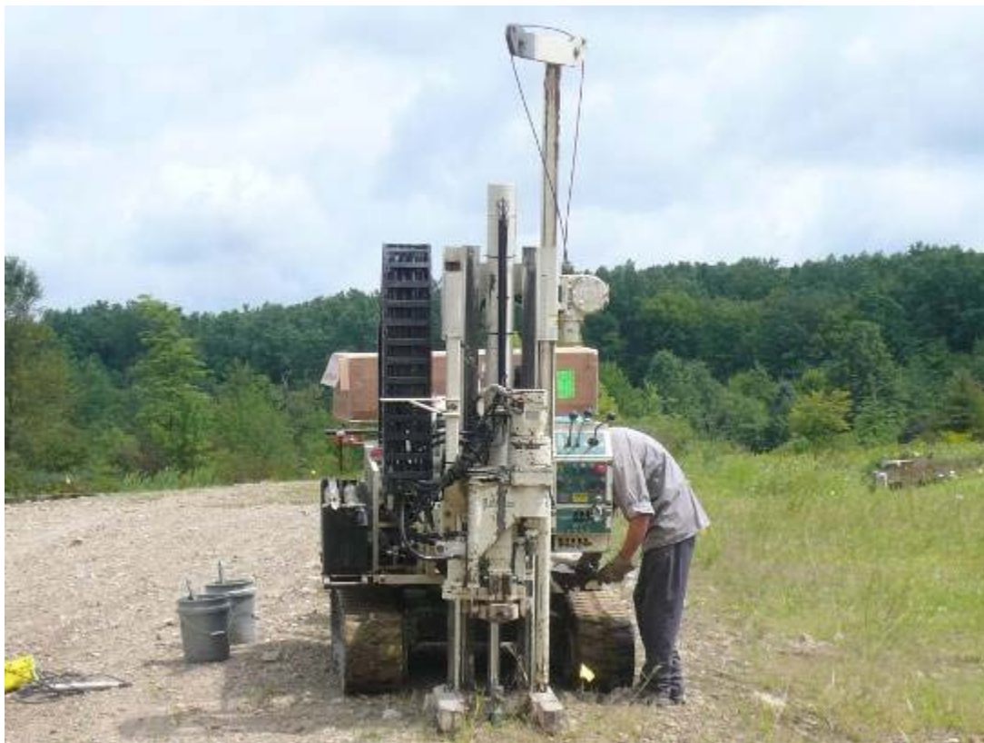
Photograph 4-5: Geoprobe Model 6620 T (Track-Mounted) Drilling Rig.
