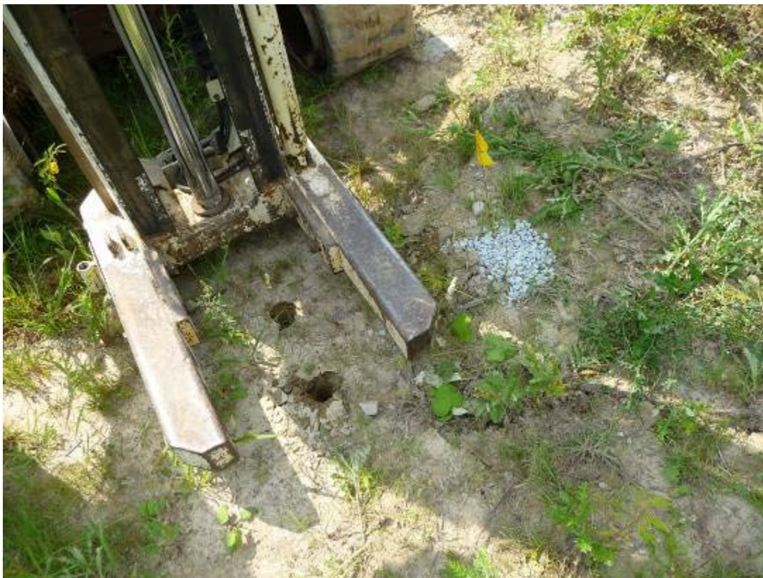
Photograph 4-9: Bentonite pellets filled all borings.
