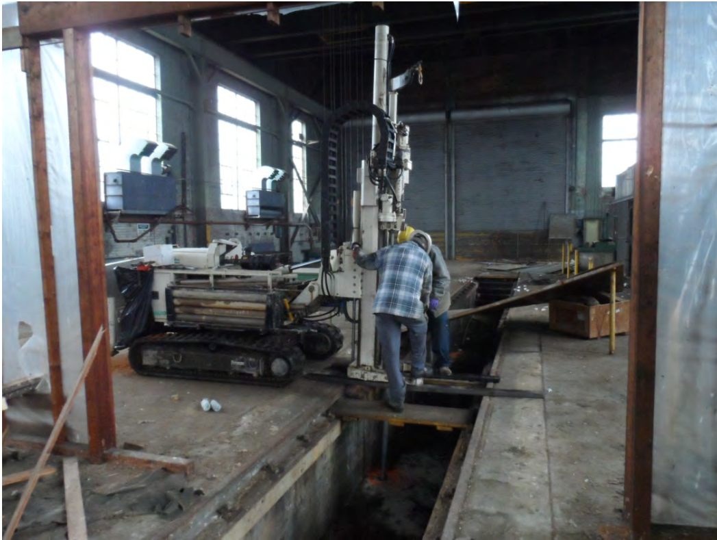
Photo 20 (2012): Direct push boring activities at the interior repair pit (DU04) within Building 47-40.
