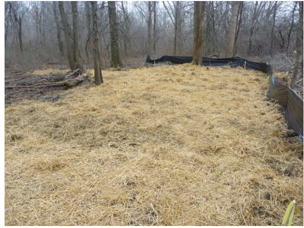
Photograph 7-2. Excavation Area after Backfill, Seeding, and Mulching
