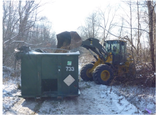
Photograph 6-2. Loading Contaminated Soil into Roll-off Box
