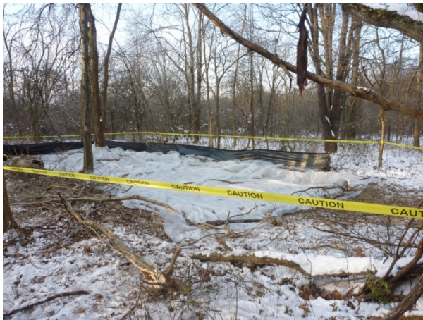
Photograph 6-3. Covered and Secured Excavated Area Upon Completing Soil Removal
