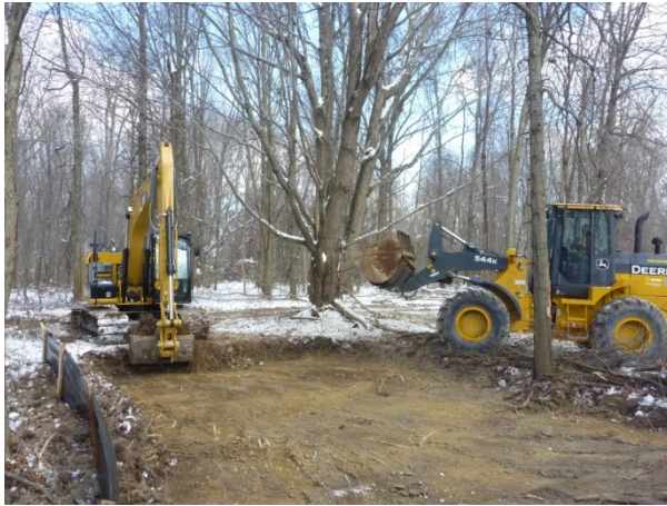
Photograph 6-1. Removing Surface Soil from Anchor Test Area
