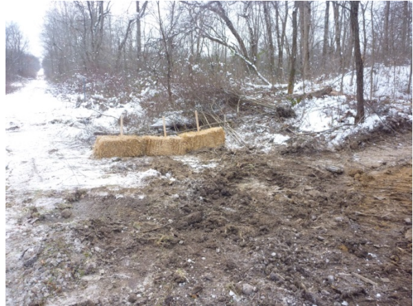
Photograph 5-2. Straw Bale Check Dam Paralleling Wilcox-Wayland Road
