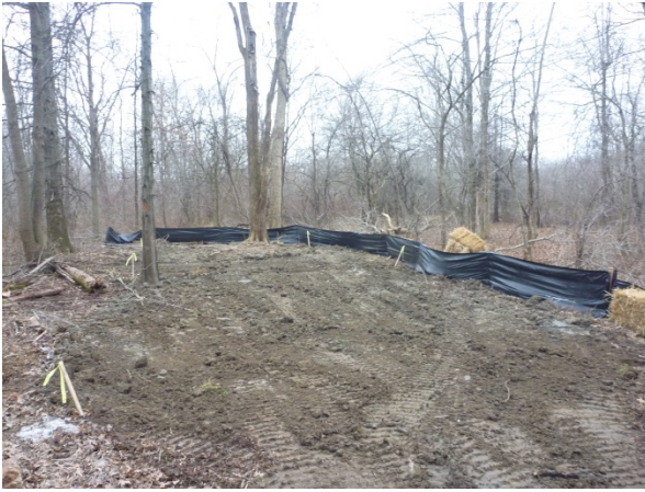
Photograph 7-1. Backfilled Excavation Area
