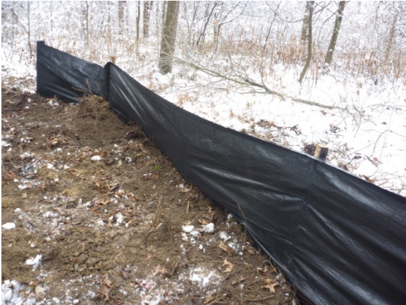
Photograph 5-1. Silt Fence Installed Downgradient of Excavation Area
