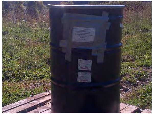
Photograph 5-10. Containerization of an Estimated 200 lbs of ACM
