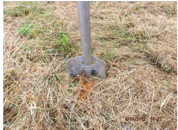
Photograph 5-8. Tubular Post Anchors
