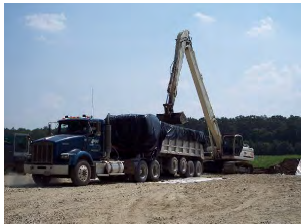
Photograph 3-8. Loading Contaminated Soil into On-Road Haul Truck
