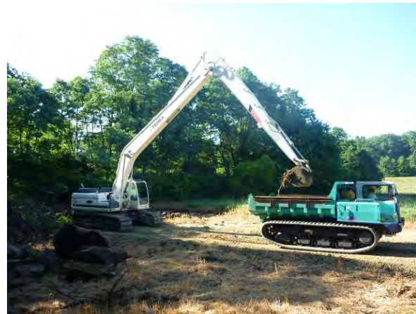
Photograph 3-4. Loading Off-Road Haul Truck
