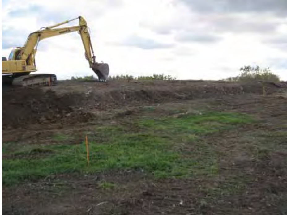
Initiating cut in berm south of Pad 61.
