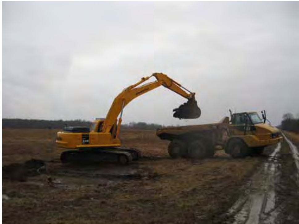
Over-excavating Pad 67 area (i.e., excavation at sample points WBG-071 and WBG-401).
