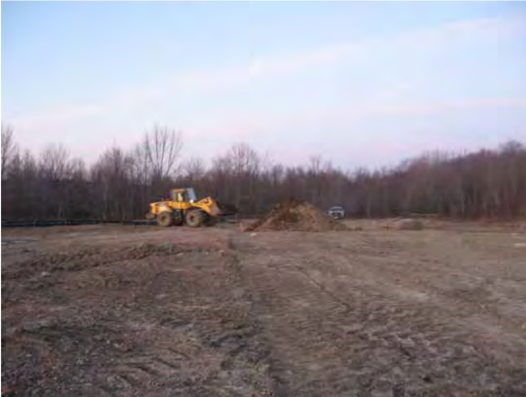
Over-excavating stockpile footprint (6-inch cut) using wheel loader.
