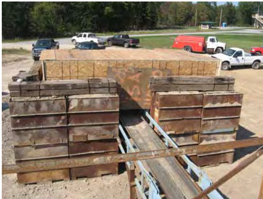
Picture showing construction of blastwall around inspection station along effluent conveyor for ferrous metal items. Similar blastwall installed at inspection station along the final soil conveyor.
