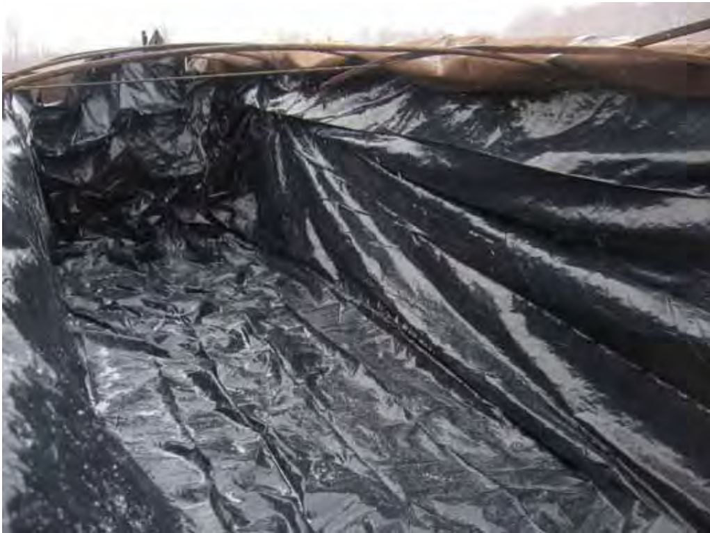
Picture showing double liner installed in truck bed prior to filling.
