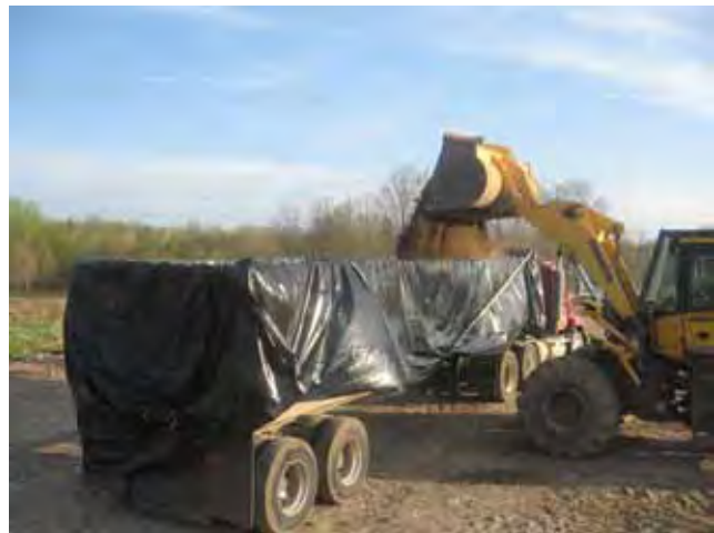
Loading out over-excavated soil from stockpile footprint.
