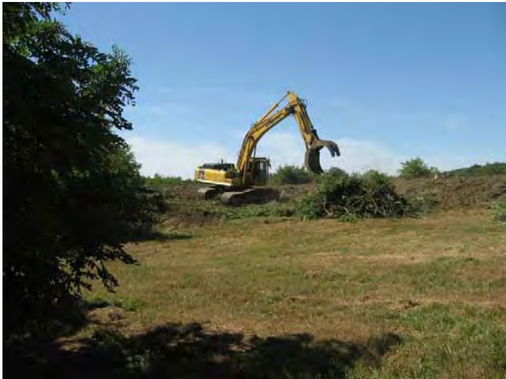
Using shielded excavator to clear heavy brush and saplings from Pads 61/61A excavation areas.
