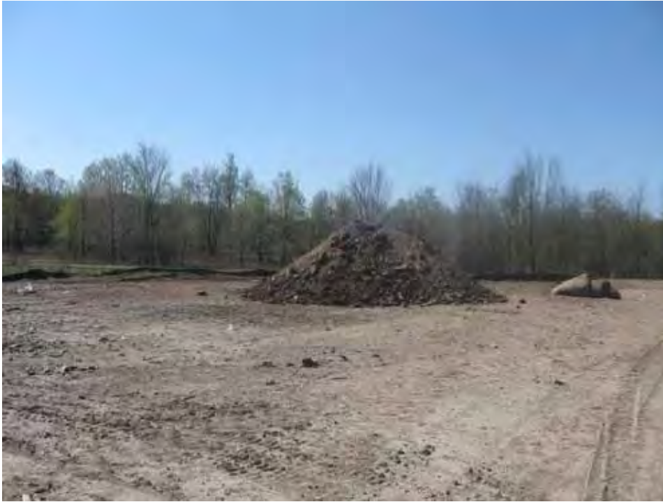
Picture showing over-excavated soil stockpile to be loaded out.
