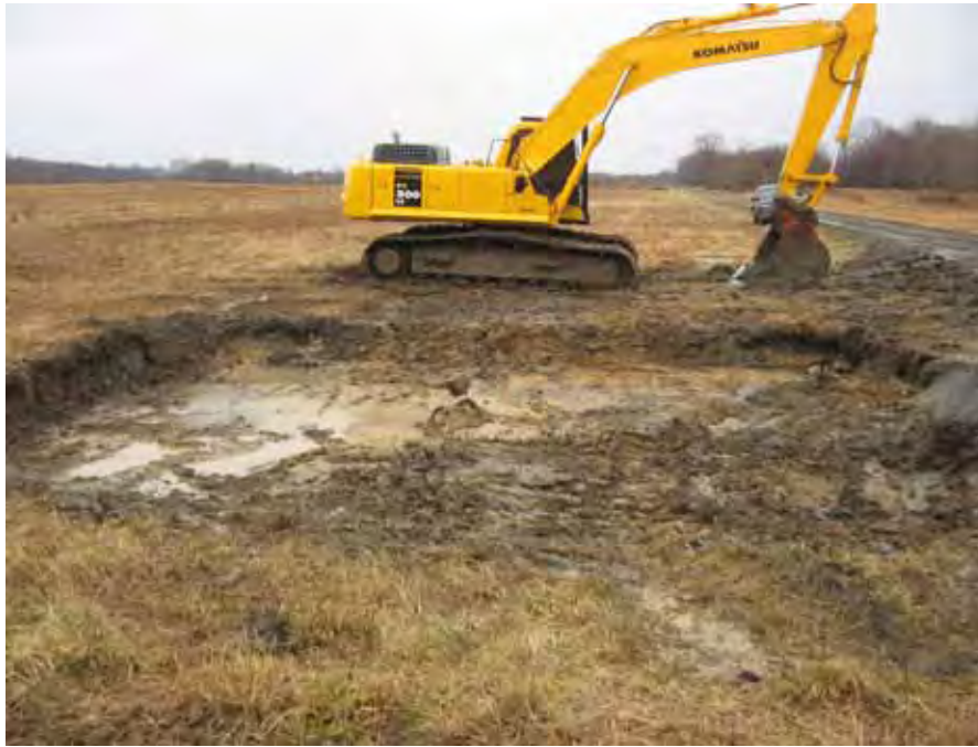
Picture showing completed over-excavation of sample points WBG-071 and WBG-401 near Pad 67.
