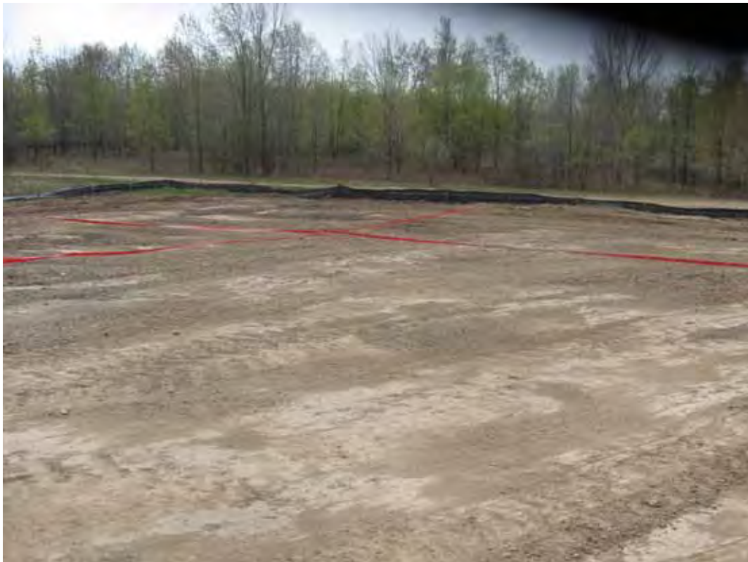
Overview of sample grids established within stockpile footprint to facilitate the sampling operations.
