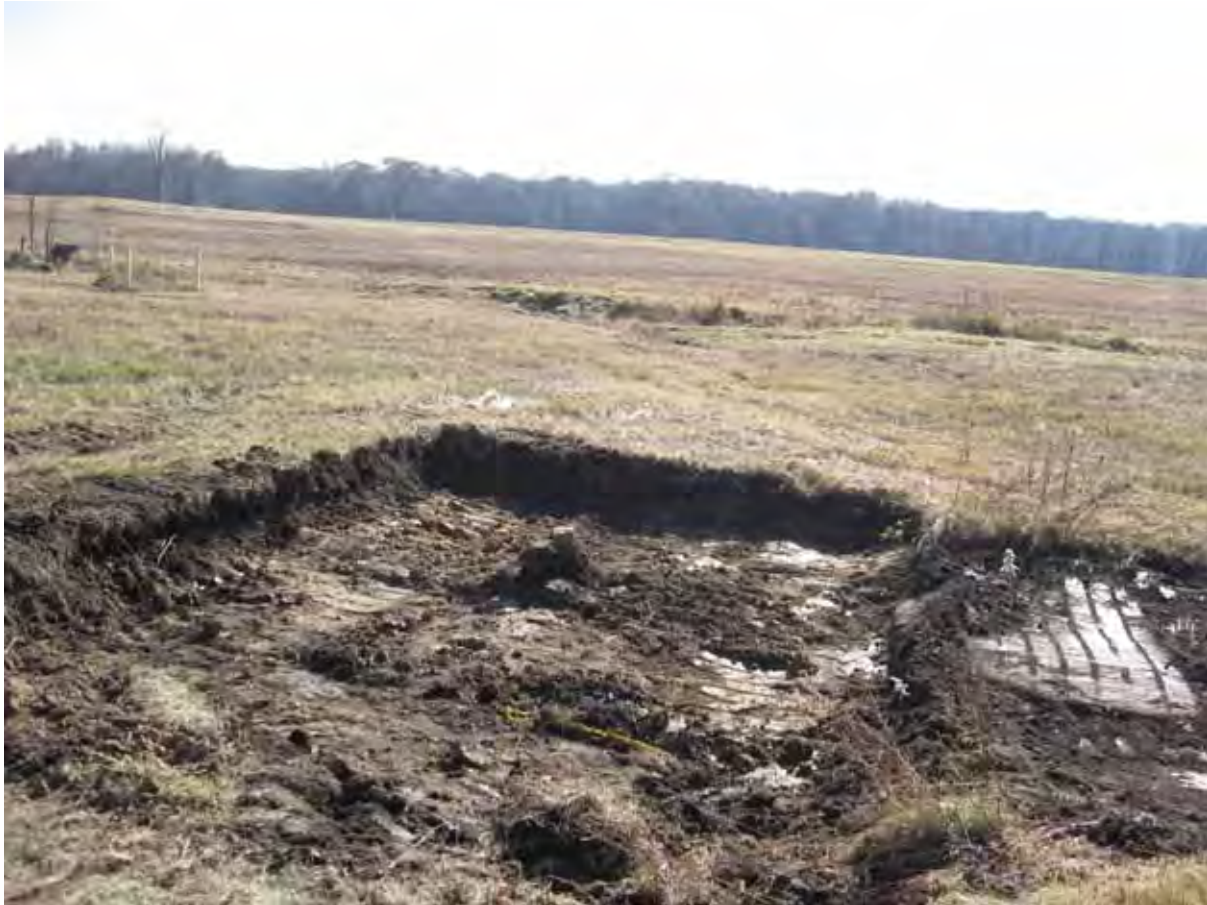
Completed “over-excavation” for sample points adjacent to Pad 67.
