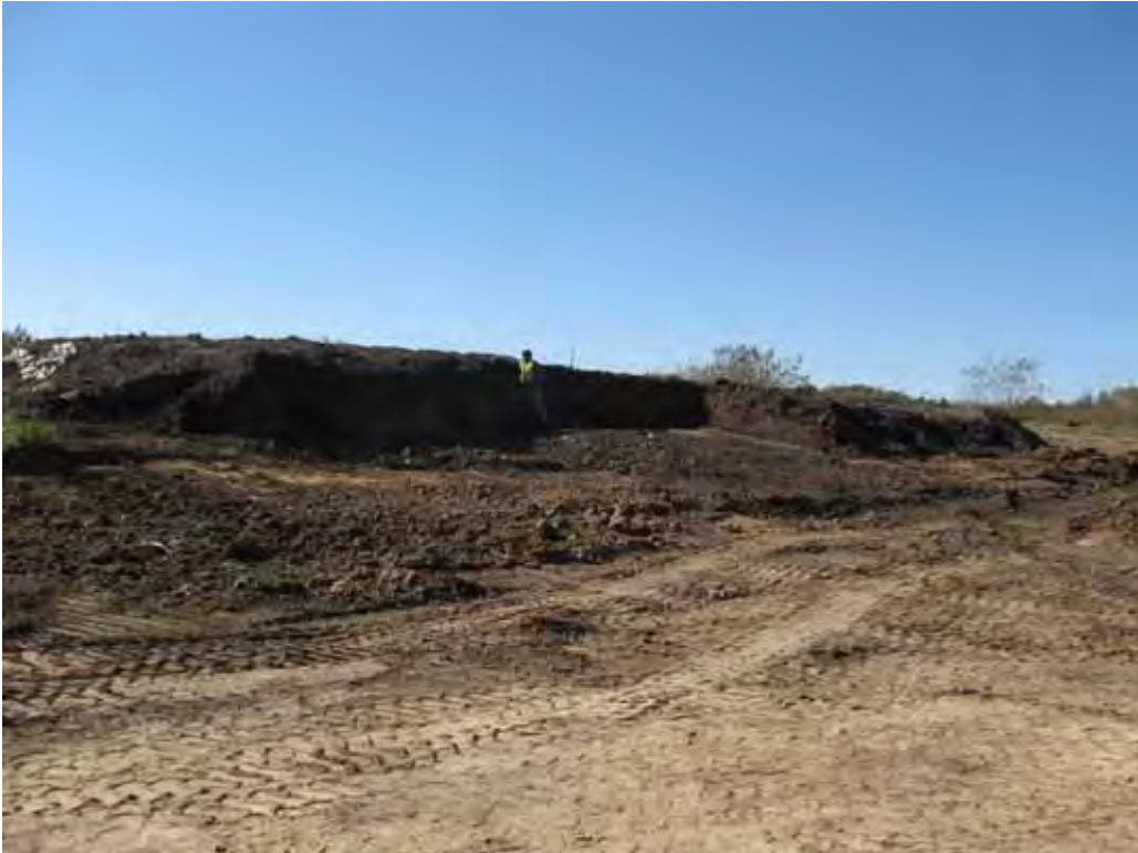
Close up of final cut in berm south of Pad 61. Notched area is the resultant over excavation area for sample point WBG-217 that was scoped for removal as par to the RA activities.
