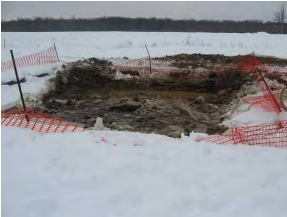
Picture showing water removed from excavation prior to sampling. Thick layer of ice removed and staged on poly to facilitate the pumping operation. Ice was returned to excavation area following sampling operations.
