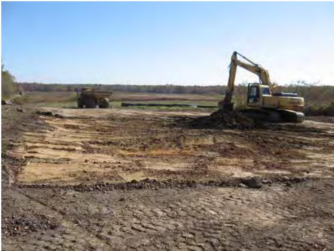
Picture showing shallow over excavation area within Pad 61A.
