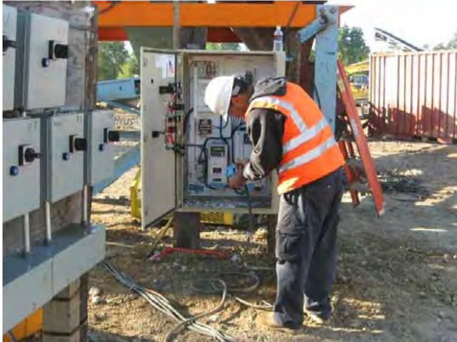
Initiating installation of control panel and power hook-ups for sift plant.
