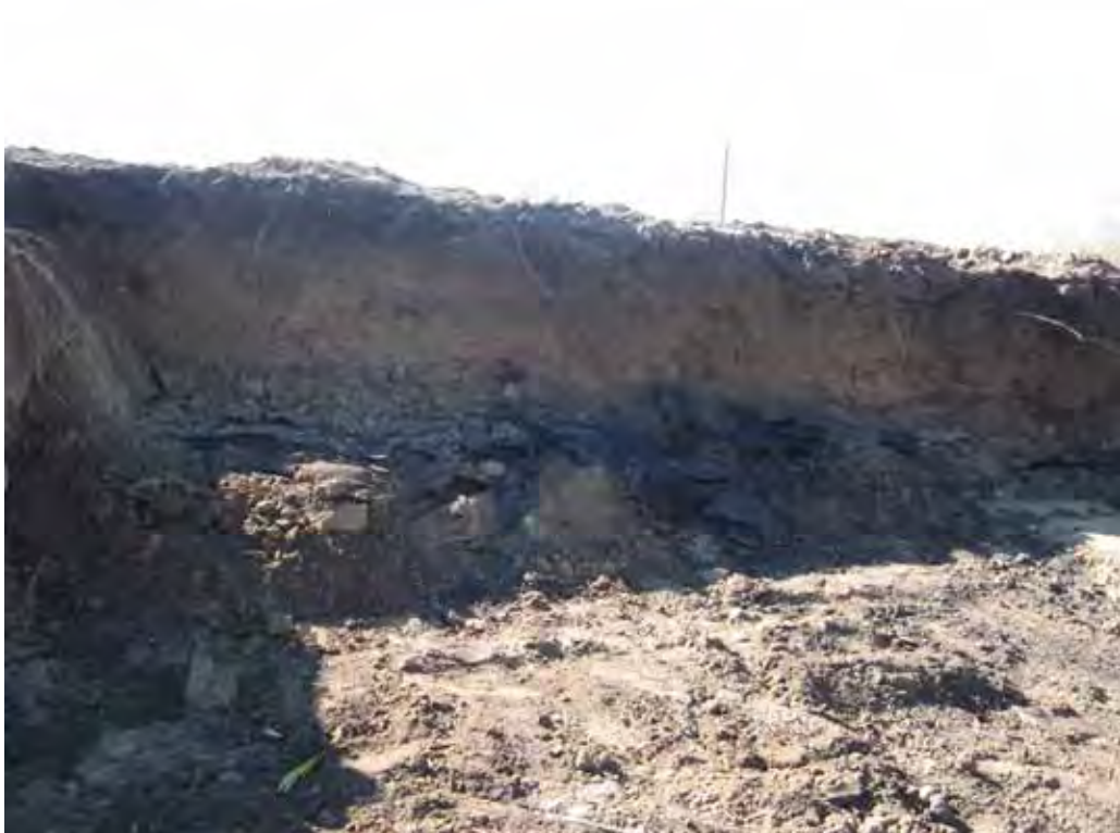
Existing layer of tar roofing shingles at limit of excavation within berm south of Pad 61.
