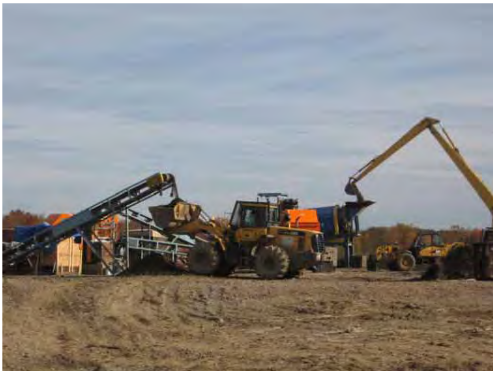
Processing excavated soil from Pad 61A. 2116 CY processed to date.
