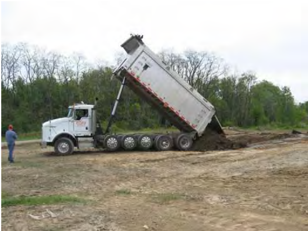
Installing back fill material for over excavated within Pad61A area.
