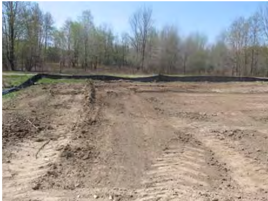
Pictures showing cross section of second over-excavation within stockpile foot print.
