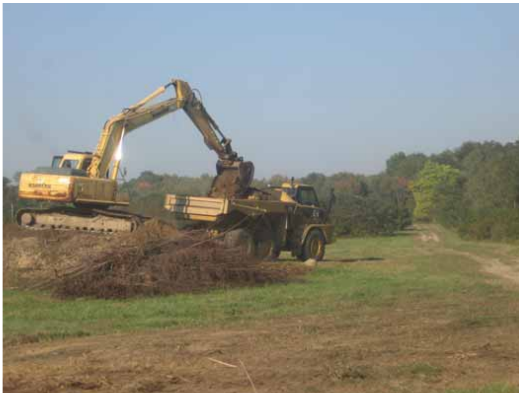
Excavating small berm on east side of Pad 61 for transport to processing area.
