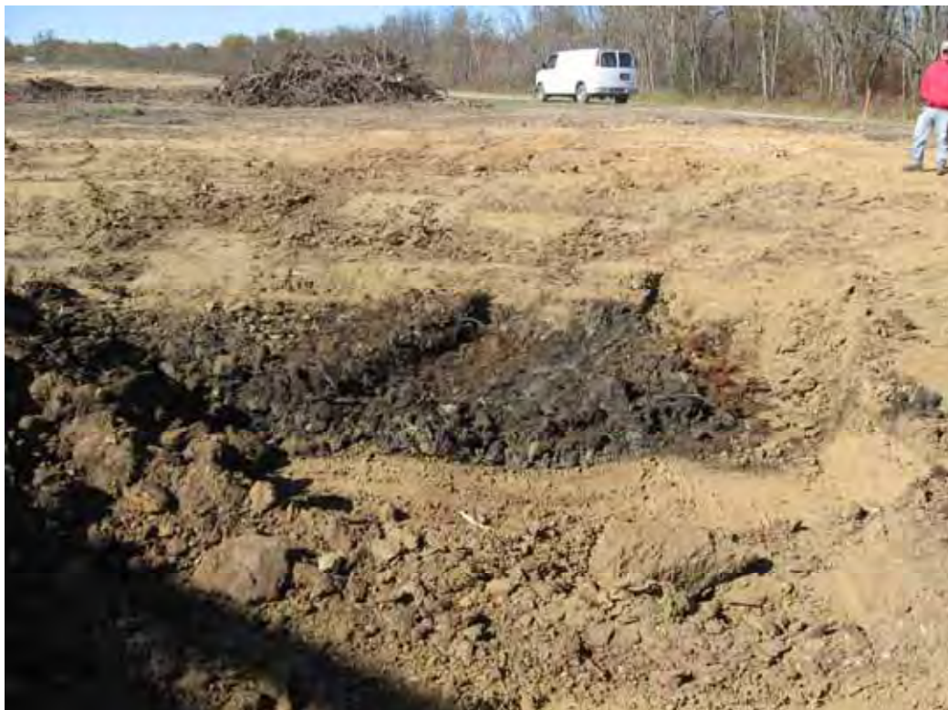
Picture showing last remaining stained area with over excavation prior to removal.
