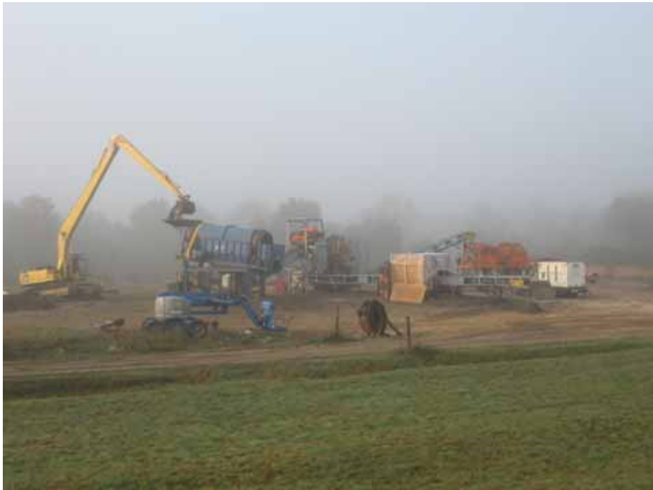
Loading excavated soil into trommel screen for processing through plant.
