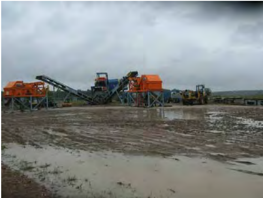
Picture showing trommel screen, ferrous magnet and eddy current magnets in place to date. Effluent conveyors and blastwalls to be installed next. Picture also showing the very wet site conditions at weeks end.
