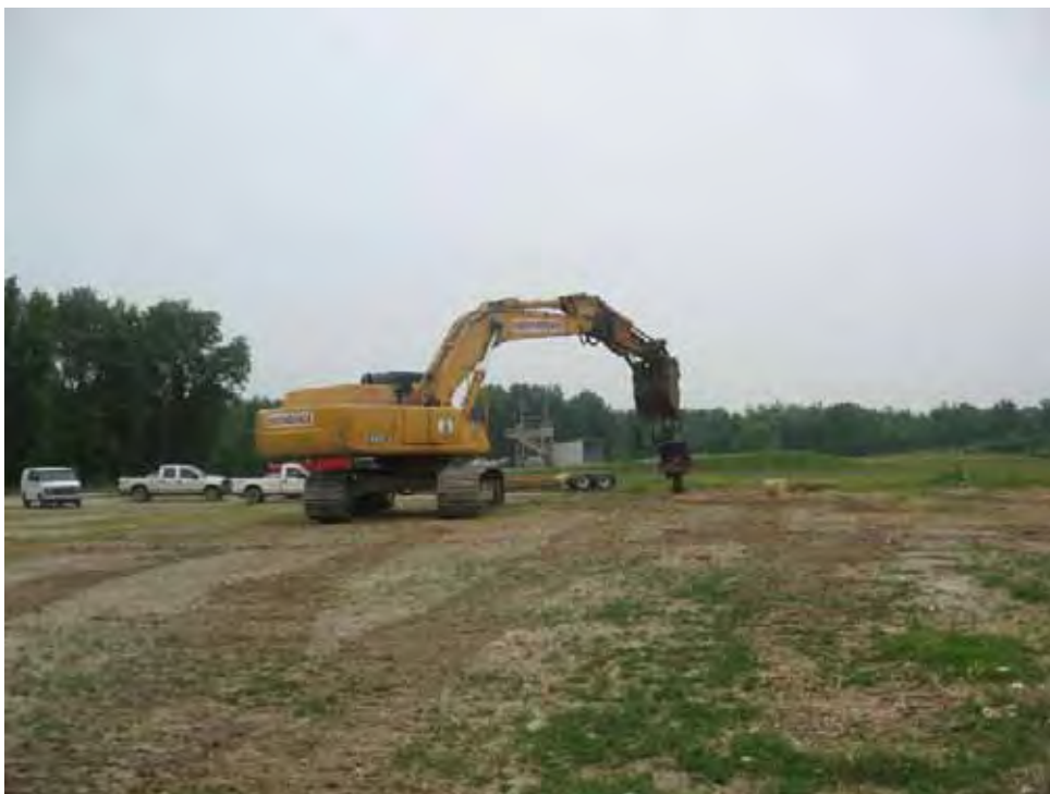
Pictures showing cleanup within process area using electromagnet.
