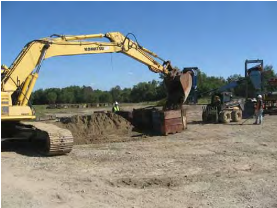
Constructing blastwalls for installation at soil and metal inspection areas.
