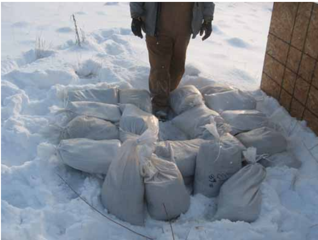
Constructing sandbag enclose for MEC demolition.
