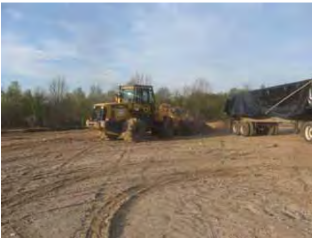
Loading out over-excavated soil from stockpile footprint.
