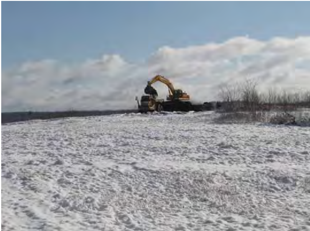
Loading out berm material for transport to processing area.
