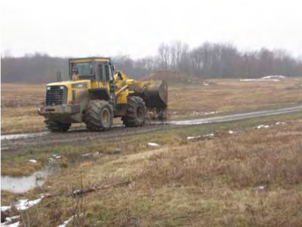
Applying ballast along eastern end of Lane C.
