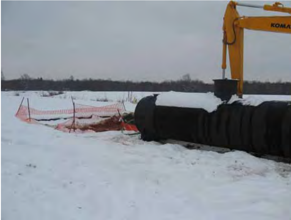
Pumping water from excavation at Pad 67 area to facilitate sampling operations. Based on sample results, water will either be discharged to the site following Ohio EPA requirements; or disposed off-site.
