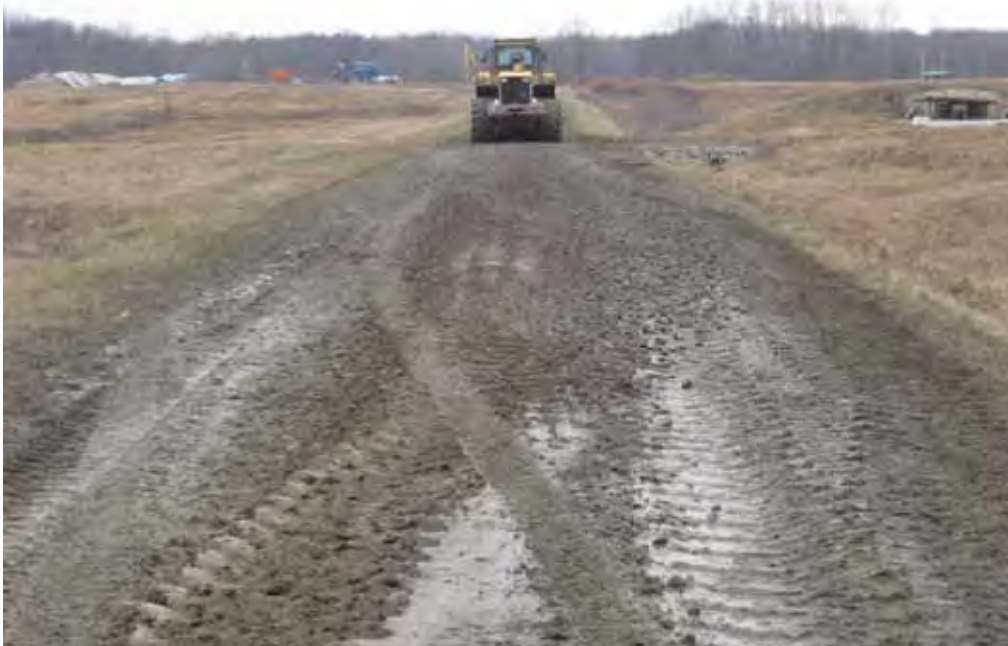
Applying initial lift of ballast along area of Lane C.
