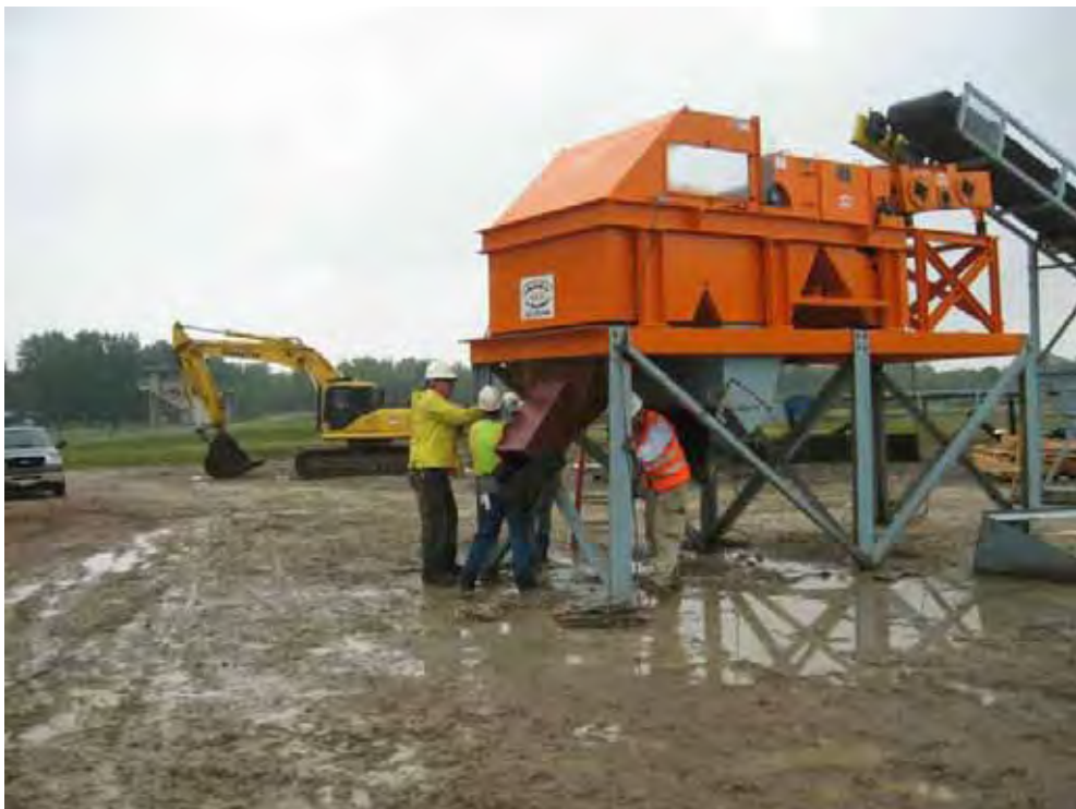
Installing chutes on eddy current magnets.
