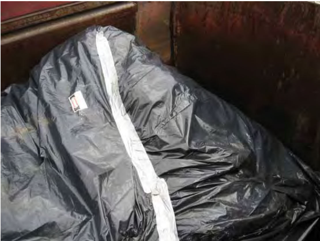
Asbestos worker securing and sealing liner for transport to disposal facility.
