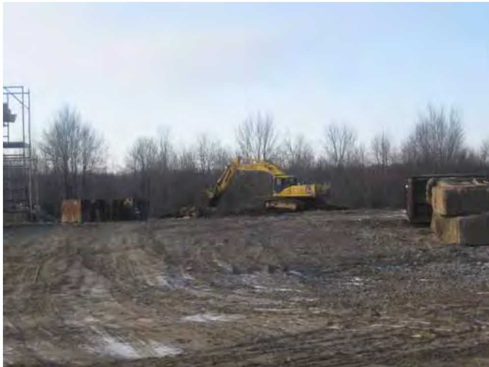
Scraping stockpile area for final clean and last loads.
