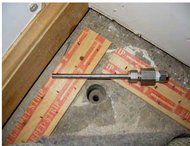
Figure 1: Assembled sub-slab port ready for installation
