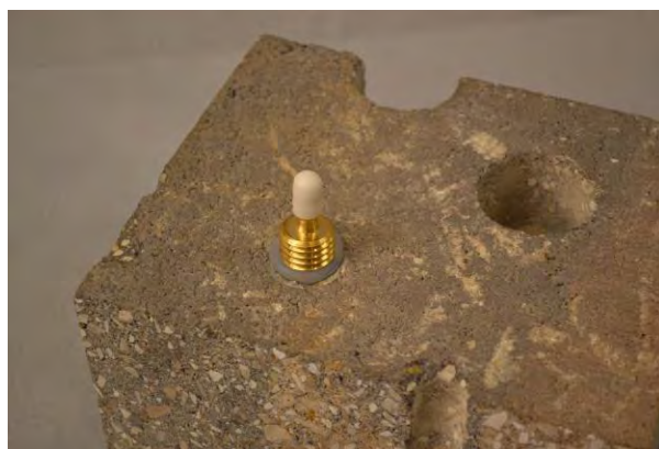
Figure 3. Installed Vapor Pin™
