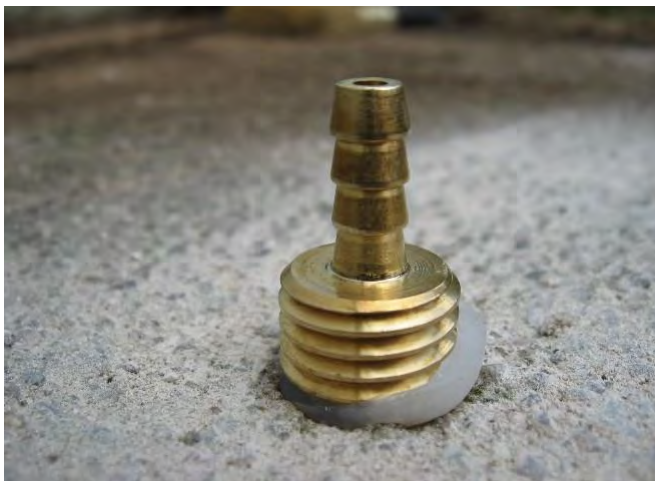
Figure 3: Vapor Pin® installed and ready for sampling
