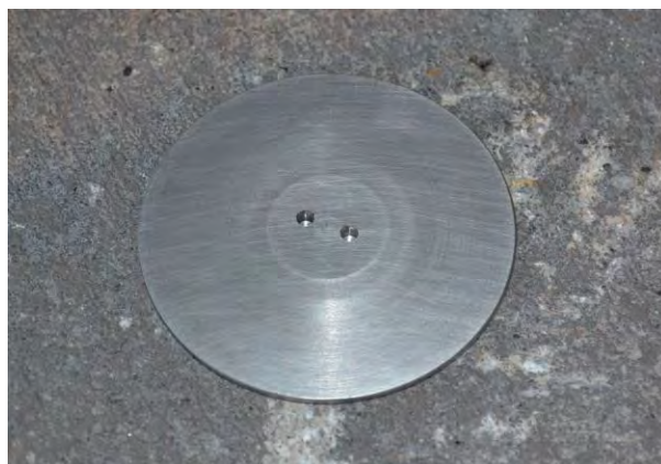
Figure 4. Secure Cover Installed
