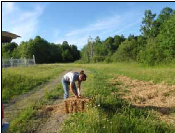
Photograph 2-9. Placement of Seed and Straw at SCFmw-004
