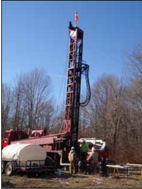
Photograph 2-5. Setup of Air Rotary Rig and IDW Polytanks on SCFmw-001
