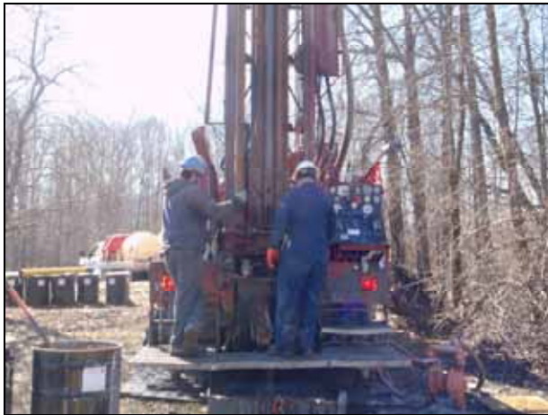
Photograph 2-7. Air Rotary Drilling
