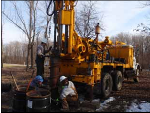
Photograph 2-3. Drilling using 12 ¼ inch ID Hollow Stem Augers
