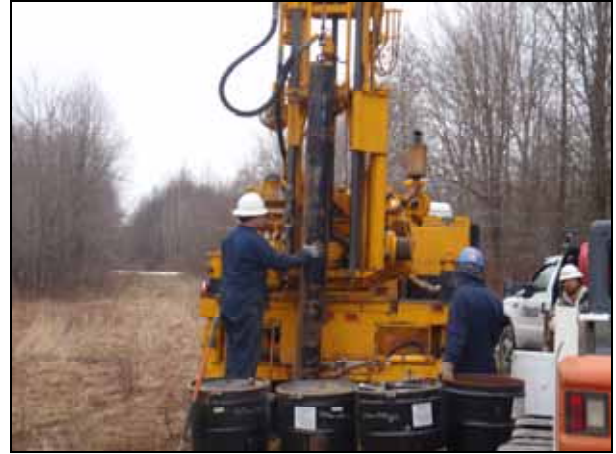
Photograph 2-4. Installation of Outer Casing through 12 ¼ inch ID Hollow Stem Augers
