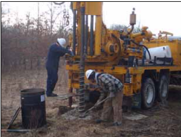
Photograph 2-1. Drilling using 4 ¼ inch ID Hollow Stem Augers
