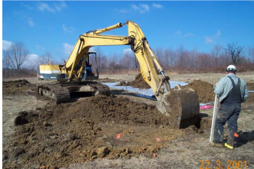
Hot Spot Excavation
