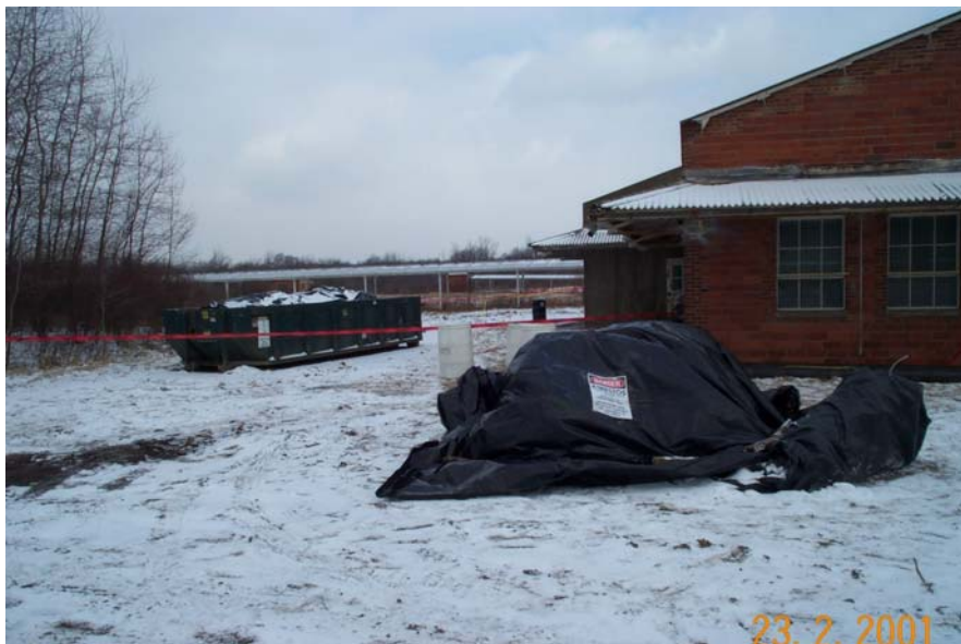
Lead Pile at AP-8
