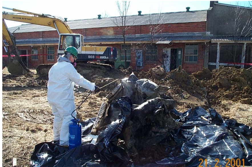
Spraying Down Lead Liner
