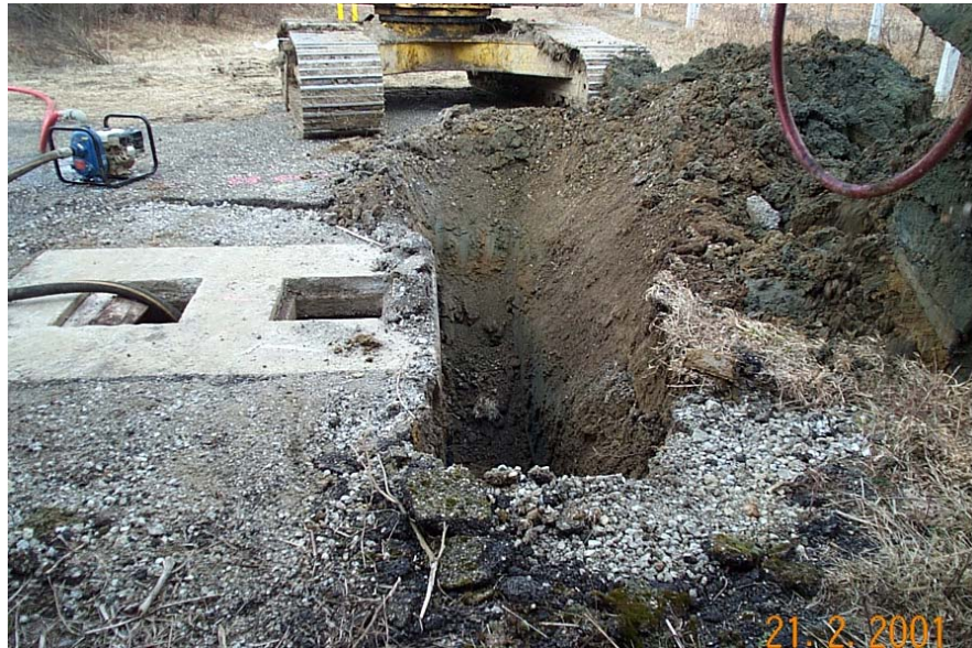
Excavating NW Sump AP-8
