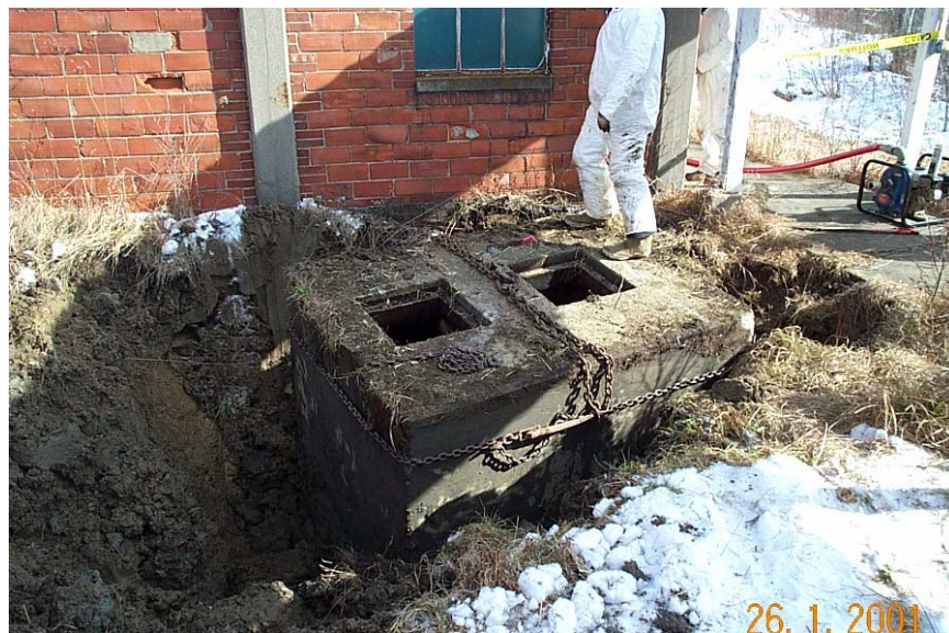
AP-5 ready to be pulled
