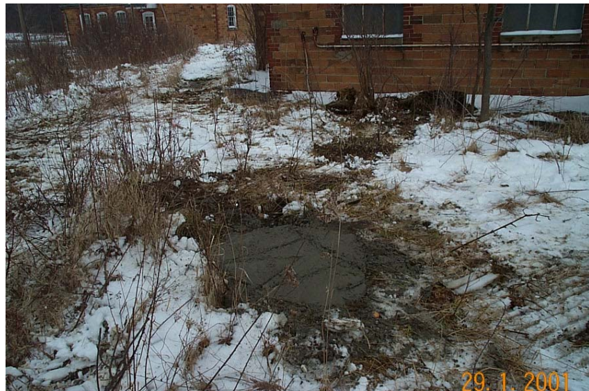
Finished Grouted Manhole
