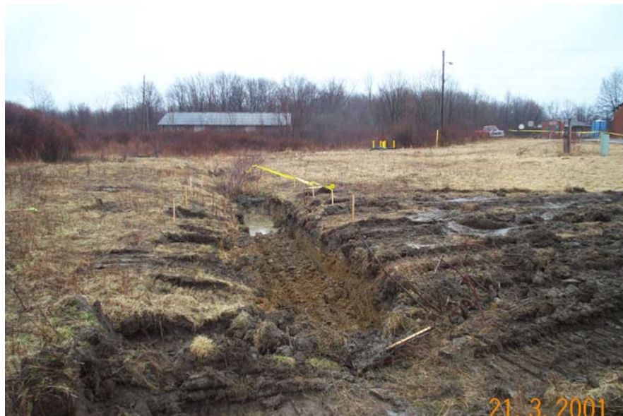
Ditch Near Gate Entry
