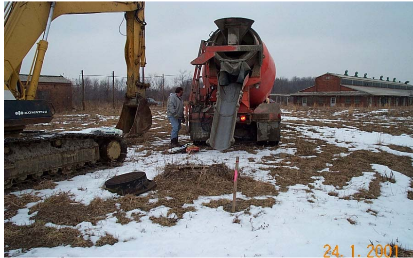
Cement/Bentonite Grouting of Manhole
