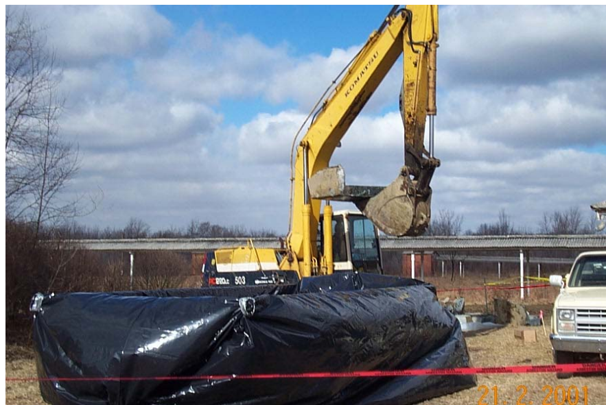
Placing Sump Cement Debris
