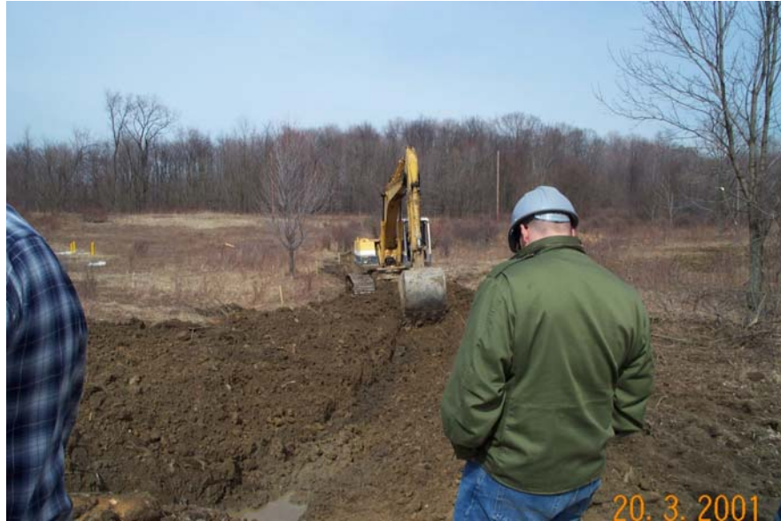
Long Ditch, Looking Away from AP-19
