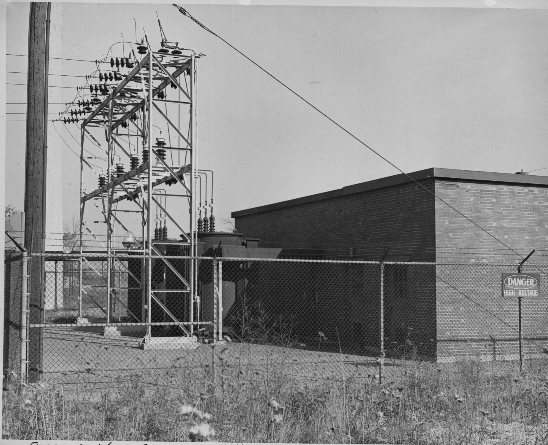
EXTERIOR - WEST SUBSTATION - REFU - RAVENNA ARSENAL
