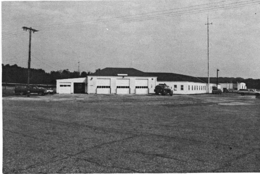
Figure 322. Building 1048: Fire House with Quarters.
