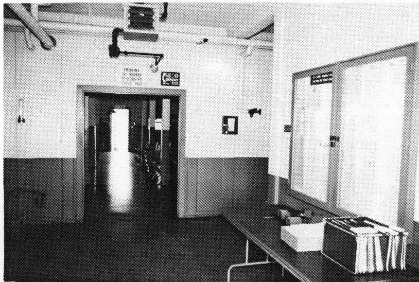
Figure 323. Building 1048A: Interior view of a Fire House with Quarters.
