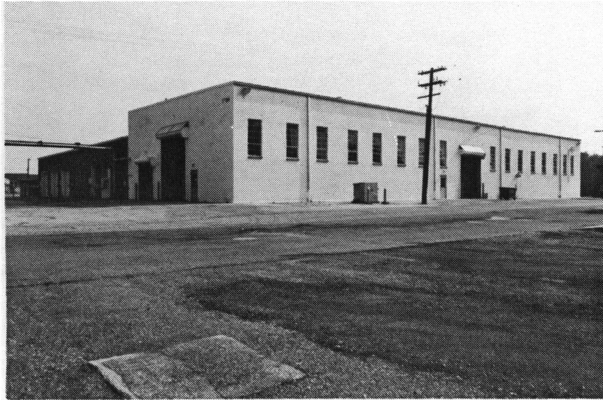
Figure 198. Building 1034: Garage and Repair Shop.
