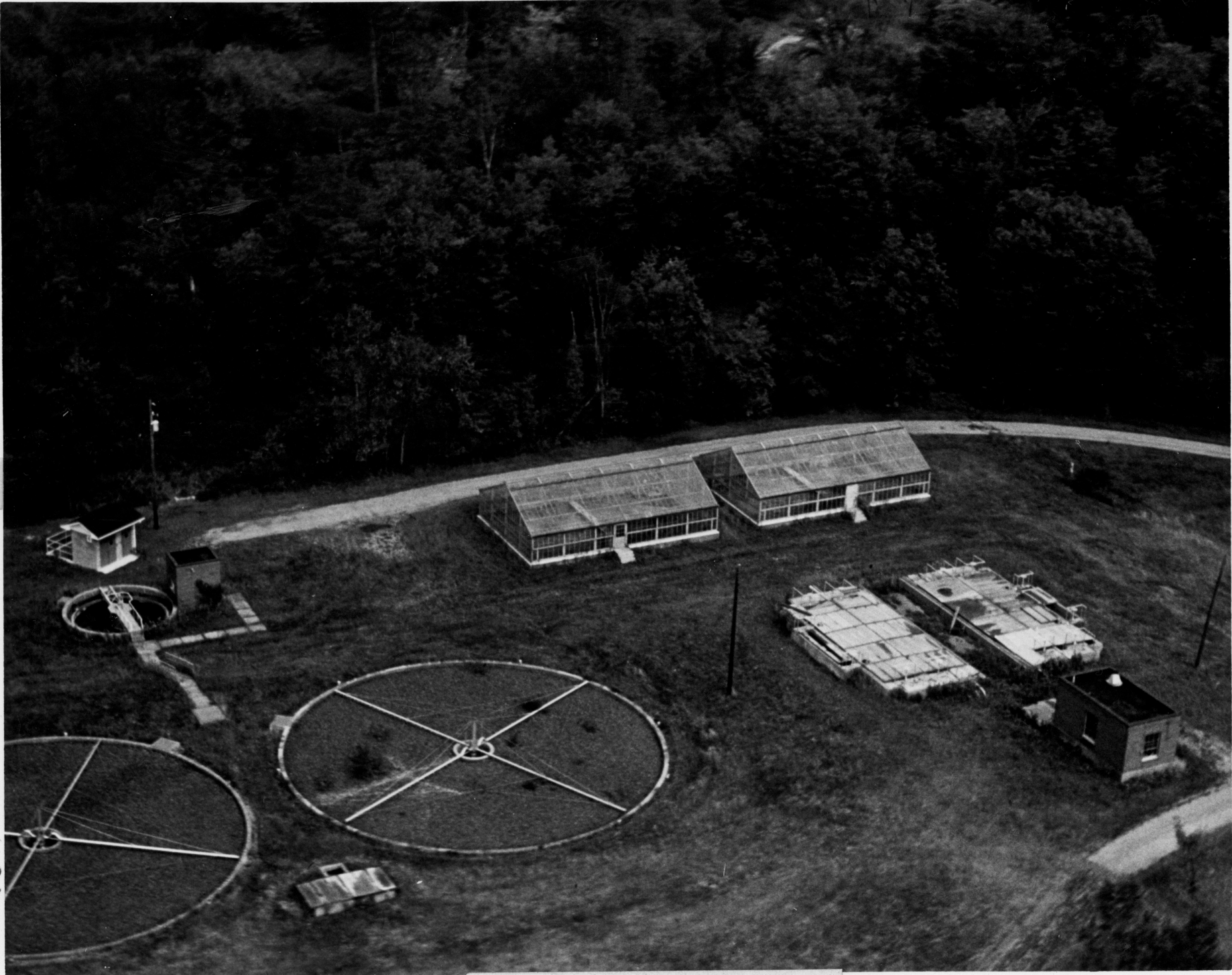
GEORGE ROAD SEWAGE TREATMENT PLANT
