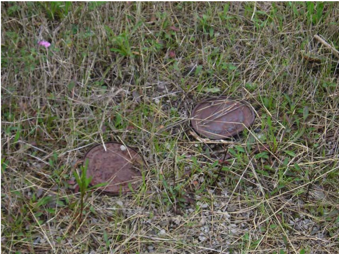
Photograph 2: Metal Lids at Site 1.
