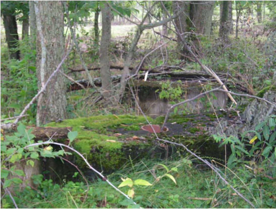
Photograph 7: Concrete pads at Site 2.
