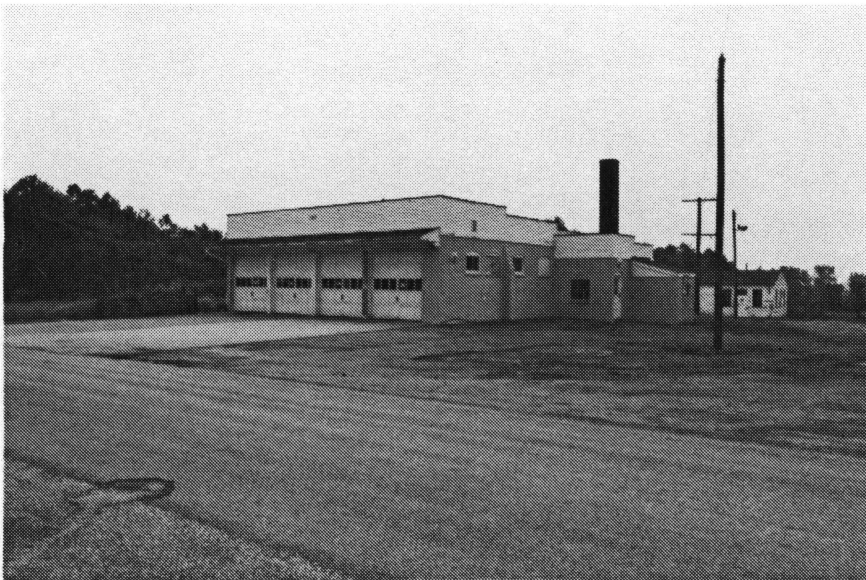
Figure 325. Building 1103: Fire House on the south service road.
