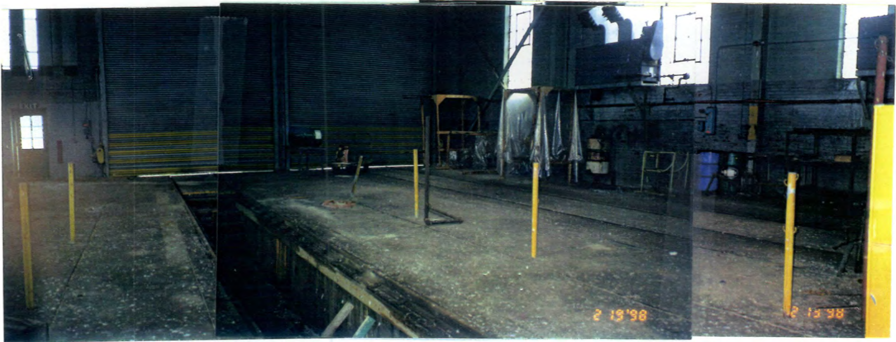
INSIDE BLDG 47-40 LOOKING NORTH
