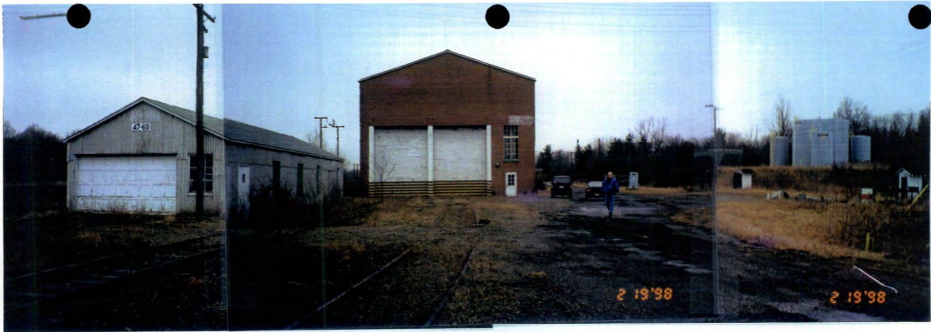
LOCOMOTIVE SERVICE BLDG- 47-40 VIEW LOOKING SOUTH
