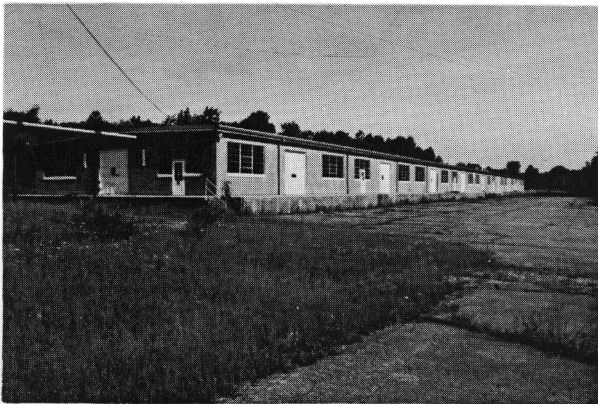
Figure 284. Building U-14: Dunnage Building.
