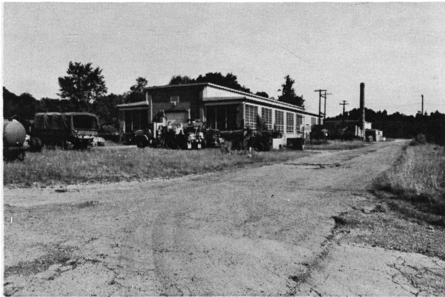
Figure 219. Building U-4: General Purpose Maintenance Shop.
