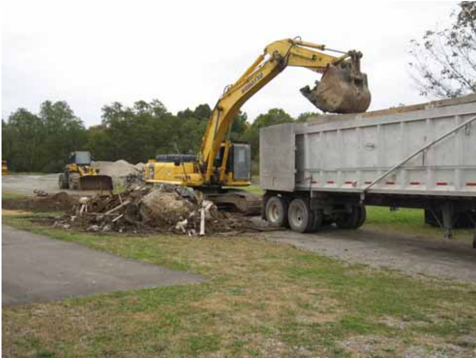
Loading out demolition debris from Laundry Flame Proofing Building.
