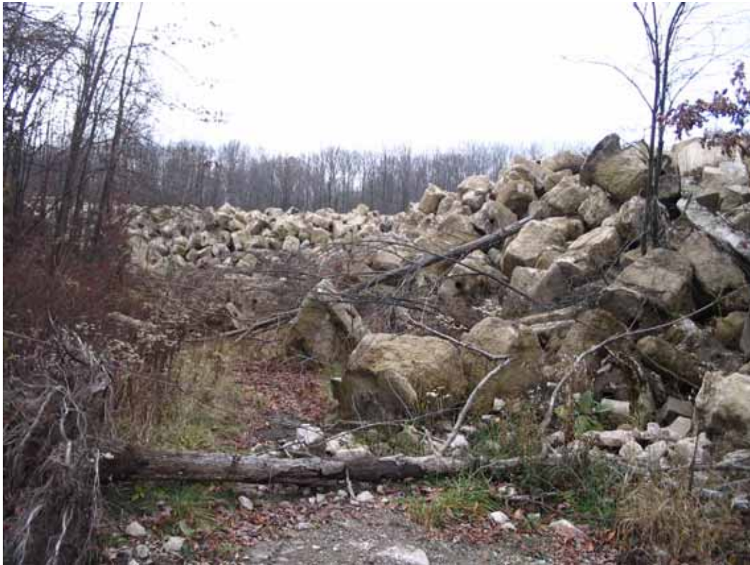
Close-up view from bottom (Change House Alley area) of CB22 Clean Hard Fill Site after fall foliage has gone.
