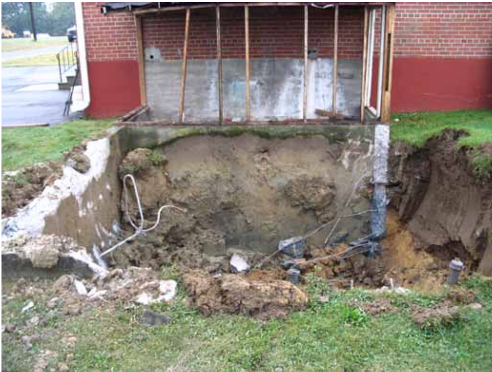
View of building and sump during demolition operations.
