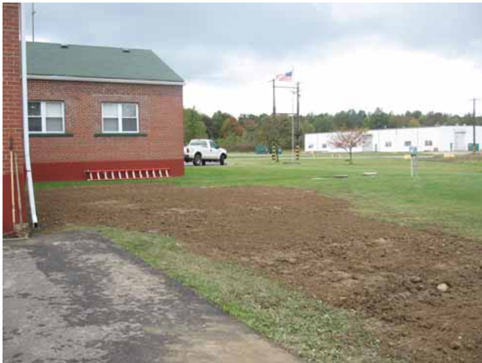
Picture showing excavation backfilled and rough graded.
