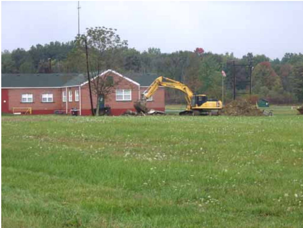
Initiating demolition of Laundry Flame Proofing Building and associated sump.
