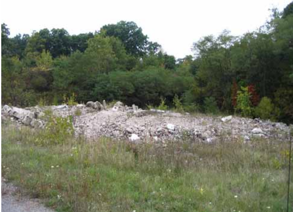
Picture showing overview of LL1 CB23 clean hard fill area.
