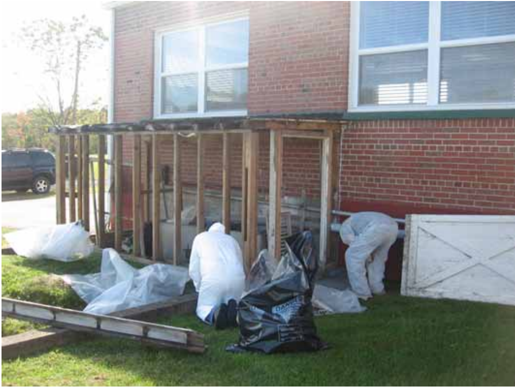
Picture showing traniste panels removed from laundry flame proofing building.
