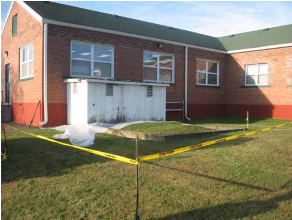
Picture showing laundry flame proofing building (small annex to brick building). Flame proofing building sump is visible in foreground.
