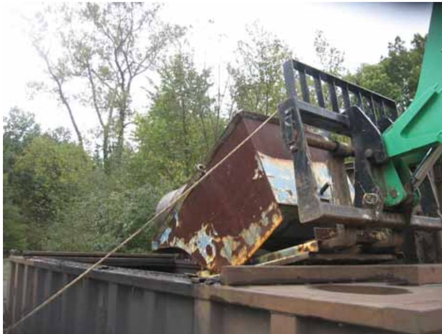
Depositing Material Documented as Safe (MDAS) into rolloff for off site recycling.
