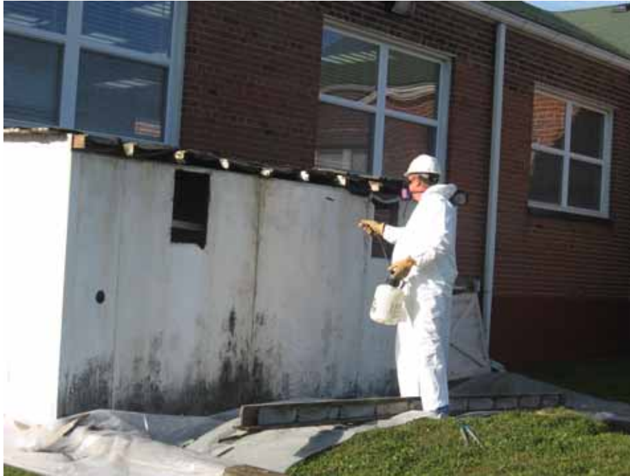
Applying amended water to traniste siding prior to removal.
