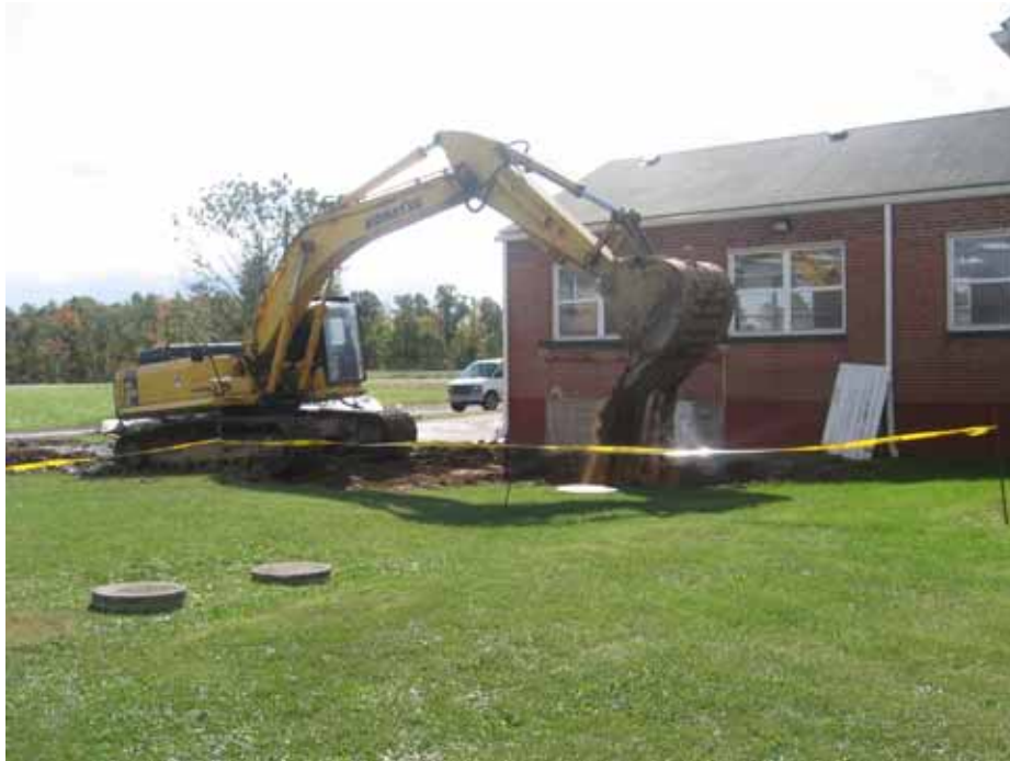
Backfilling excavation area.
