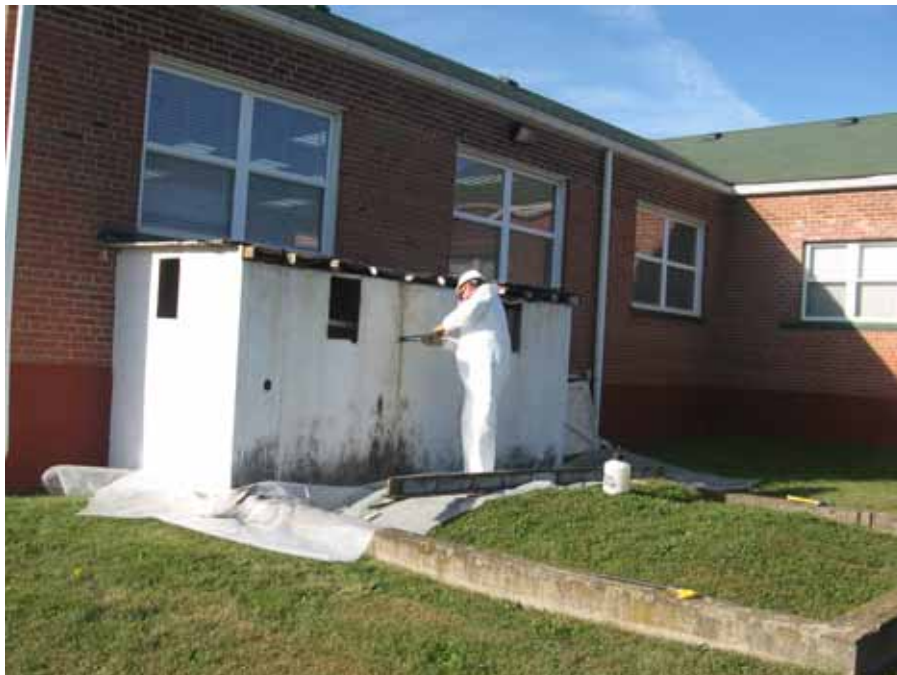
Asbestos worker removing panel bolts.
