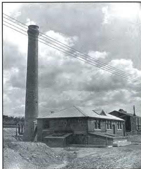
Figure 5-56d. Bundling Buildings Area power house with lunch room in background. War Department photo, RVAAP Collection
