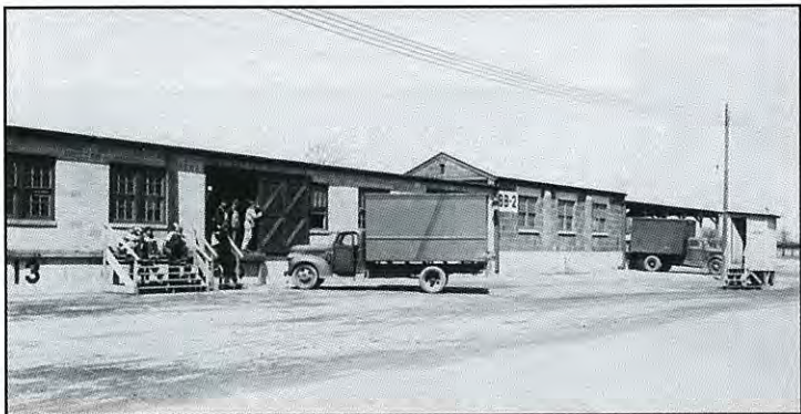
Figure 5-56c. One of the Bundling Buildings with a crew on a break and posing for the photographer. War Department photo, RVAAP Collection
