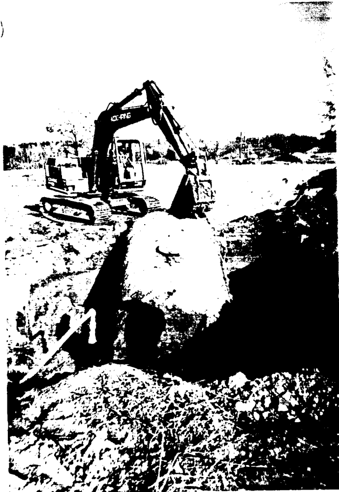
A-1 SITE REMOVAL & DECOMMISSION
