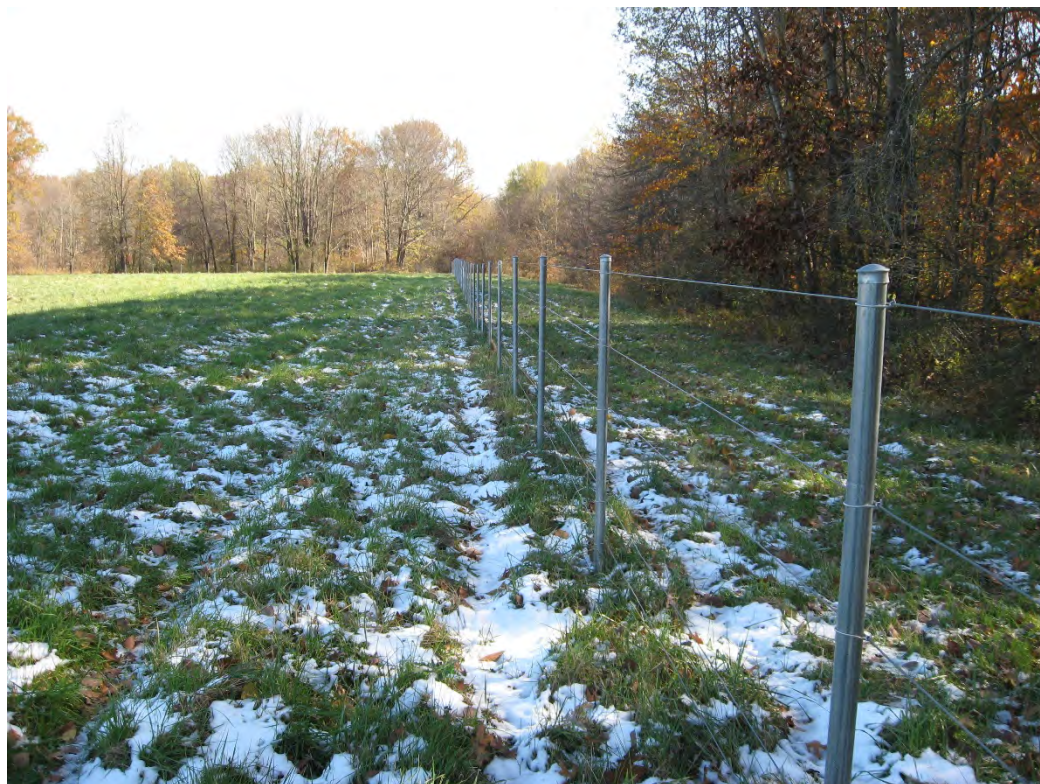
Southern 5-wire tensile fence at Ramsdell Quarry Landfill, looking east.
