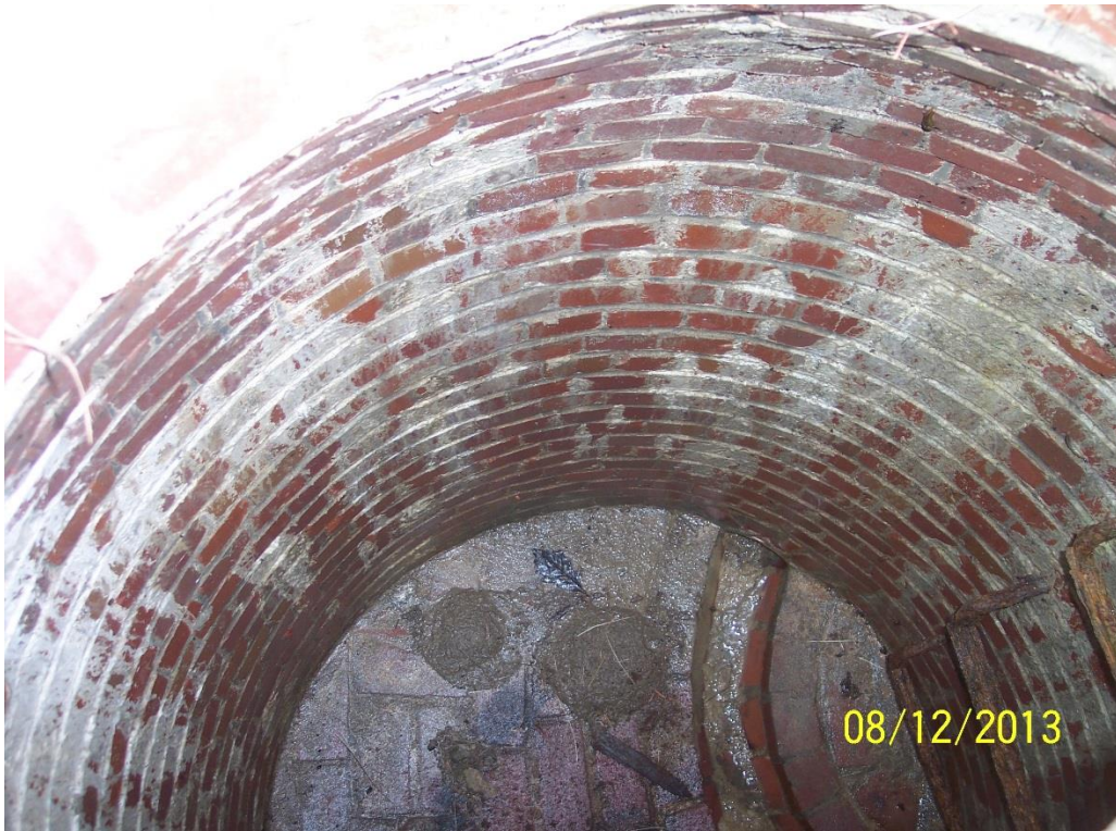
View of incoming pipe in manhole. Manhole bottom is at 7 ft bgs.
