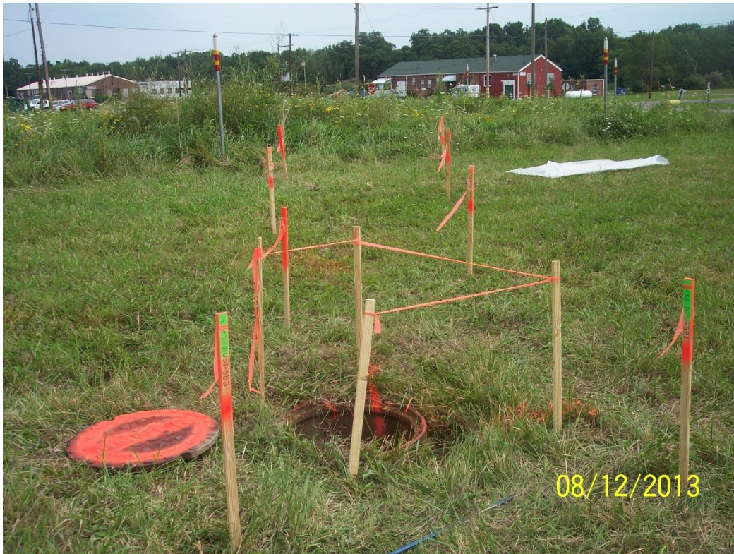
View is looking towards the northeast. Note orange paint line on edge of manhole rim. This denotes direction of incoming pipe at the bottom of the manhole.
