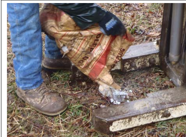
Sealing Drilling Location with Bentonite Pellets
