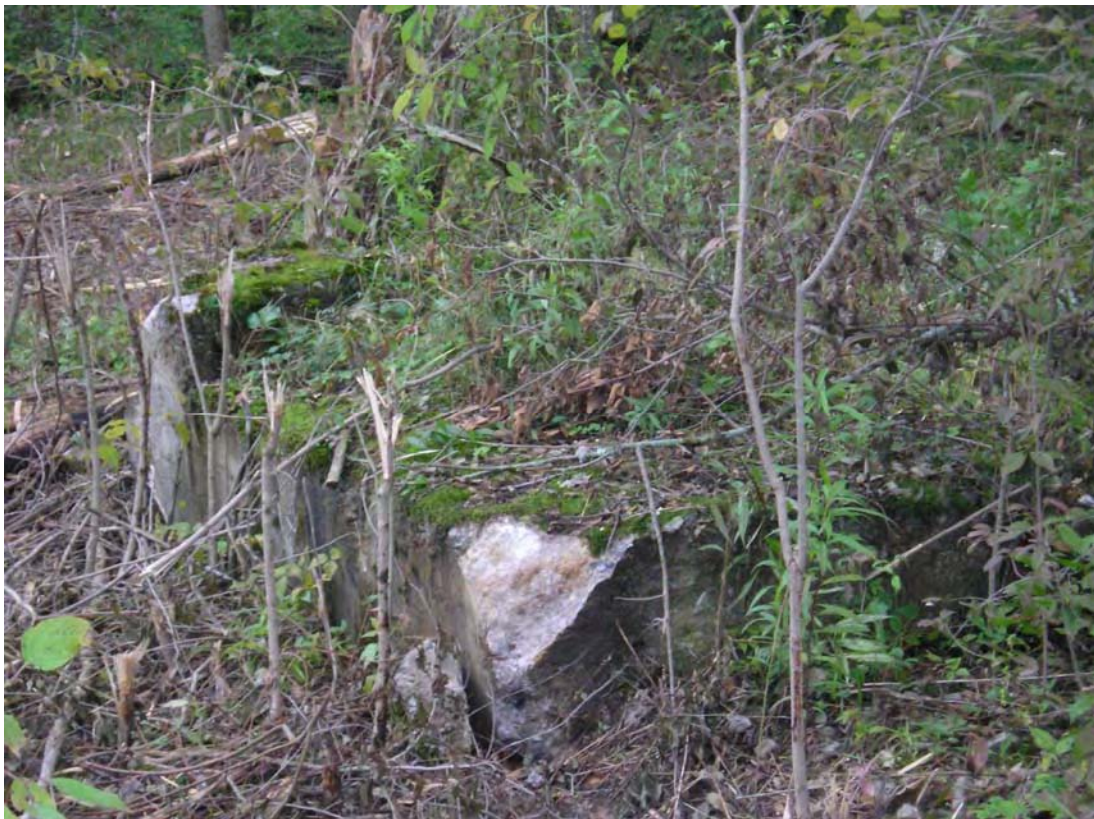
Photograph 8: Another view of concrete pads at Site 2.
