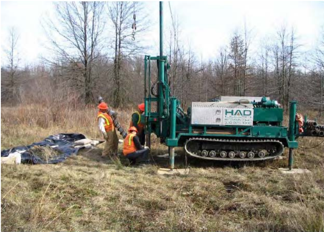
040 - ATV HSA rig on a monitoring well location at LL 12.
