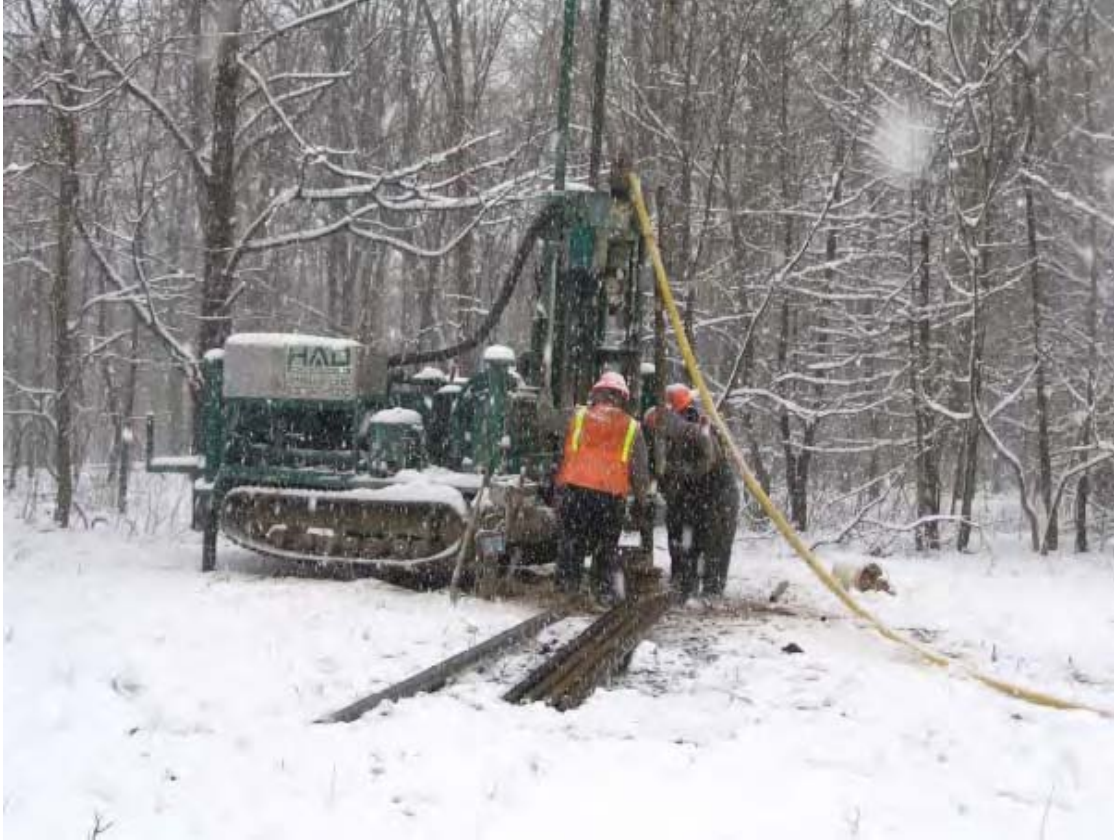
041 - Preparing to core bedrock at C-Block Quarry.
