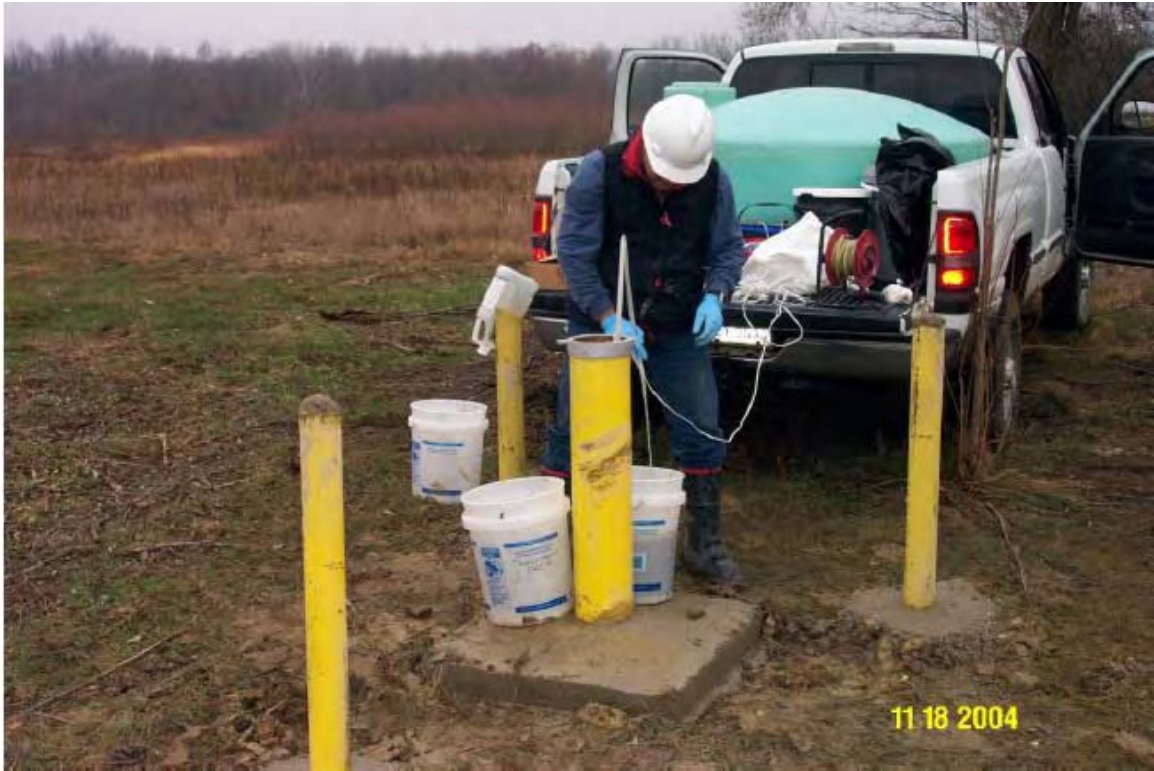
053 - Groundwater monitoring well development at Atlas Scrap Yard.
