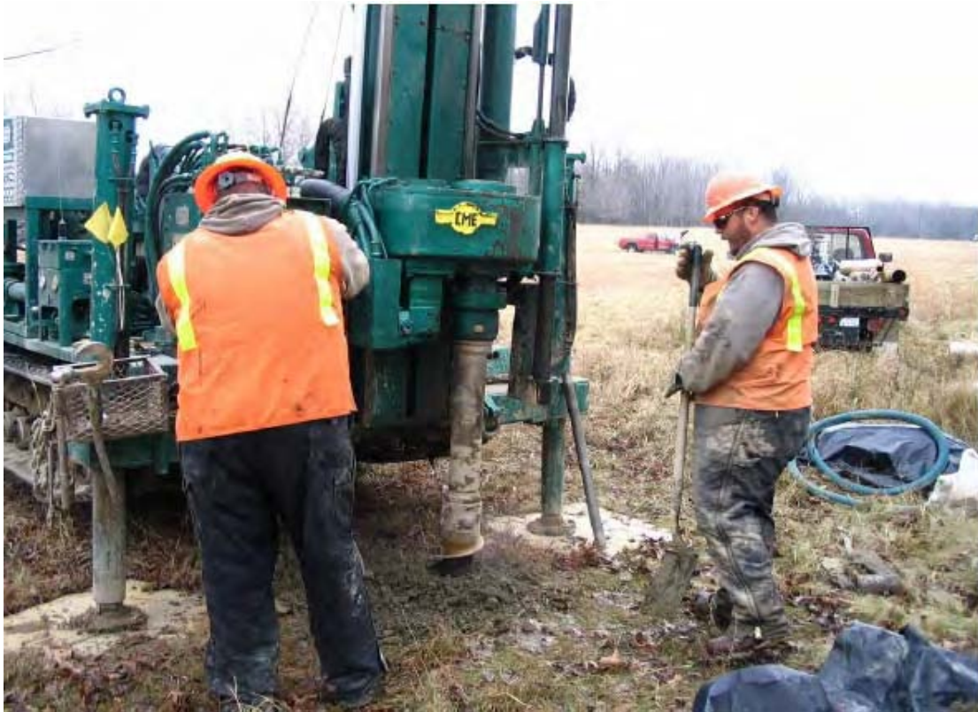
049 - Groundwater monitoring well installation at NACA Test Area.
