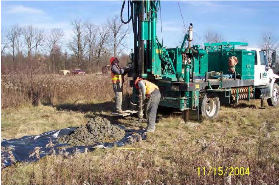
047 - Groundwater monitoring well installation at Atlas Scrap Yard.
