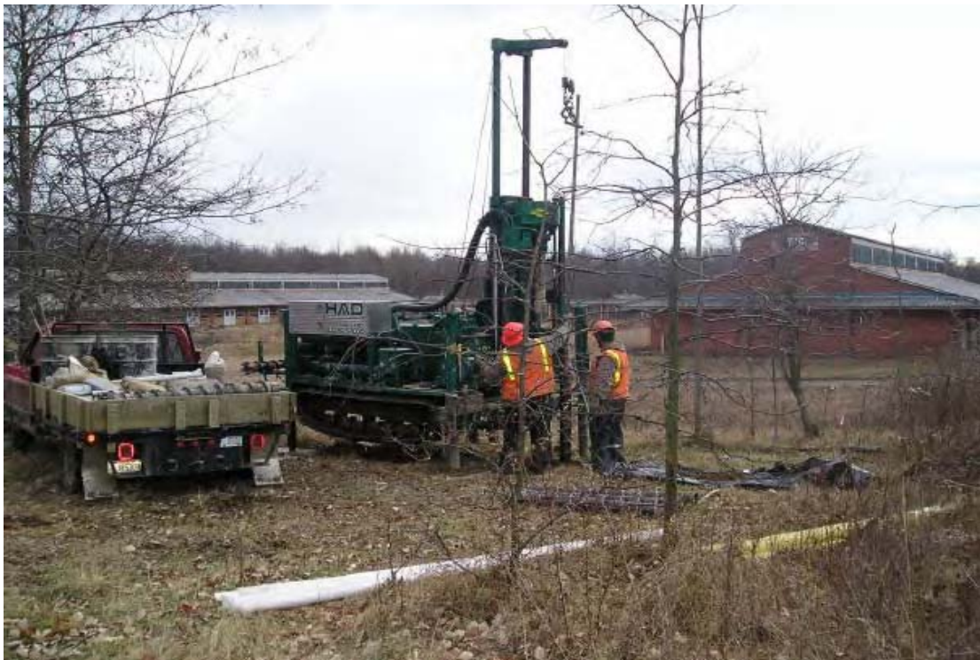
050 - Drilling operations at LL 8.
