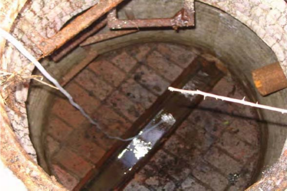
027 - Sump condition at LL 7 (water present but no sediment present).
