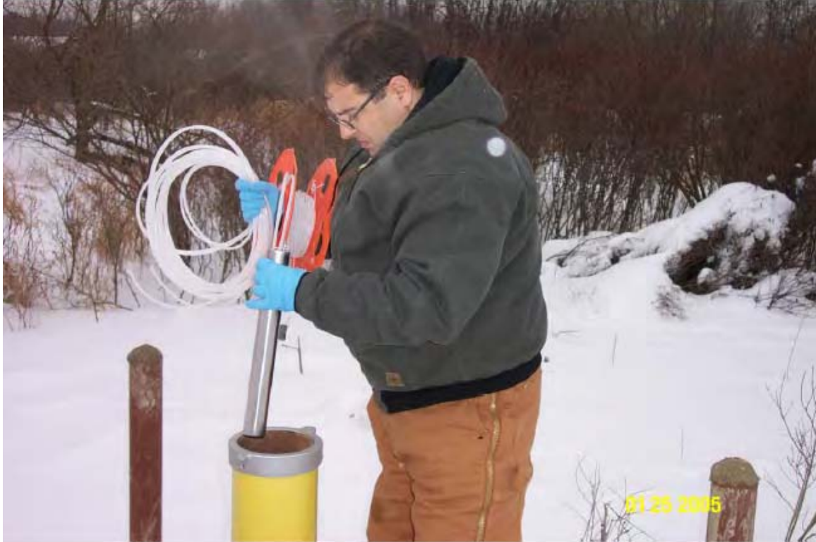
065 - Groundwater monitoring well sampling at LL 7.
