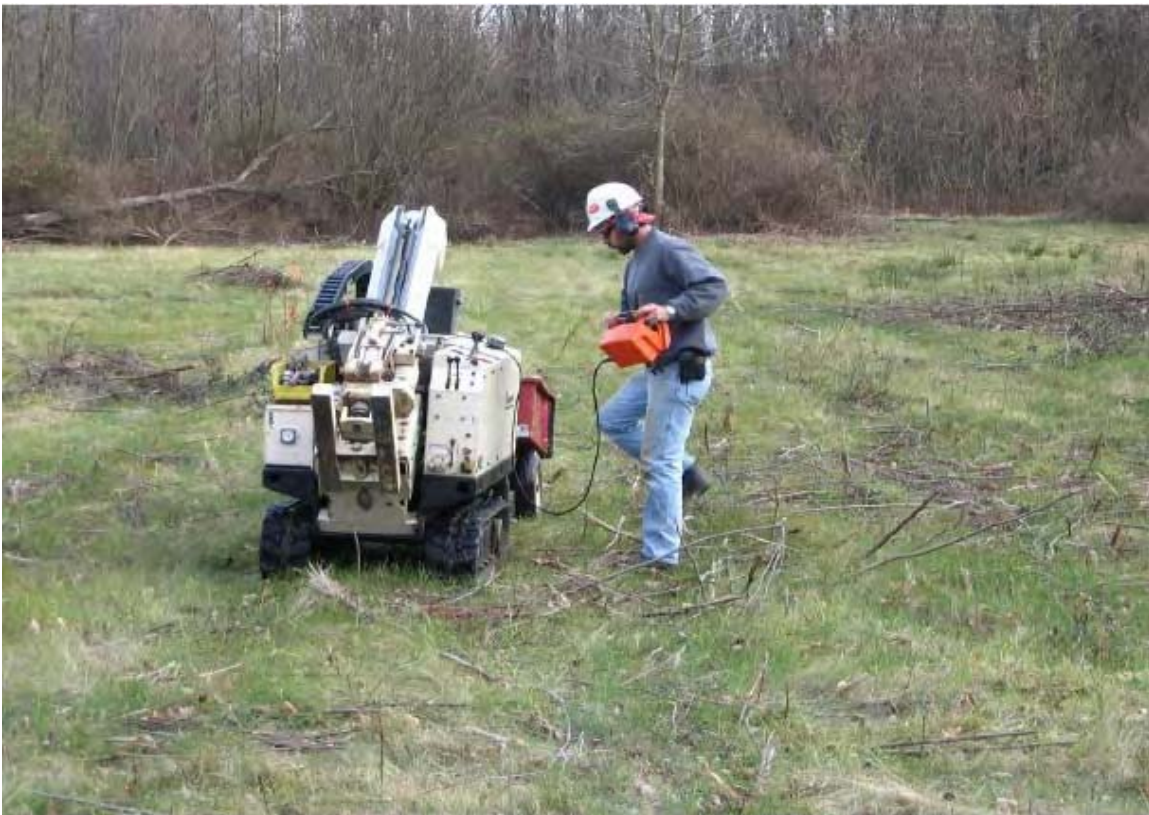
036 - Moving the ATV Geoprobe rig to a boring location at the Landfill N. of Winklepeck.
