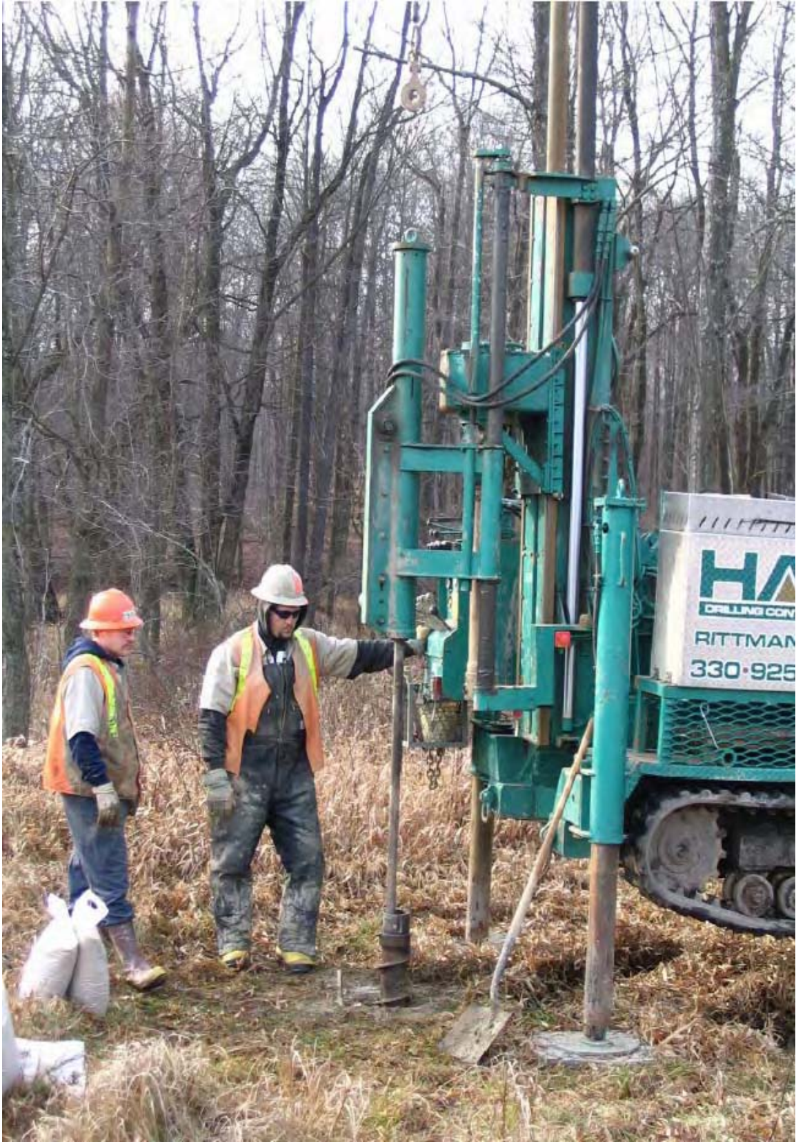
051 - Groundwater monitoring well installation at NACA Test Area.
