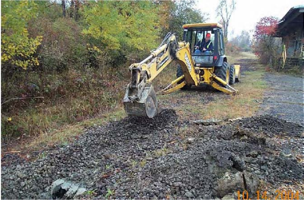
009 - Ballast removal from the railroad bed adjacent to buildings F-15/F-16
