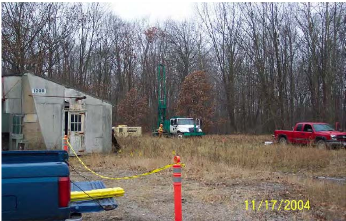
048 - Groundwater monitoring well installation at Building 1200.
