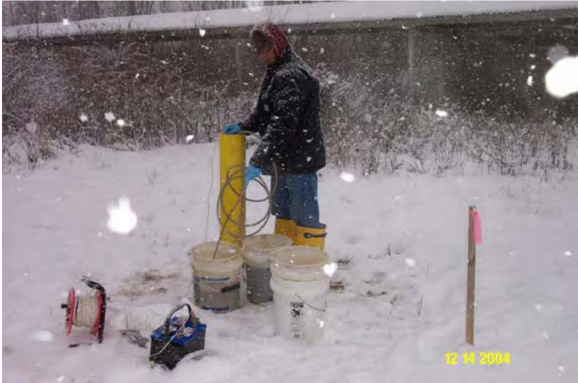
056 - Groundwater monitoring well development at LL 8.
