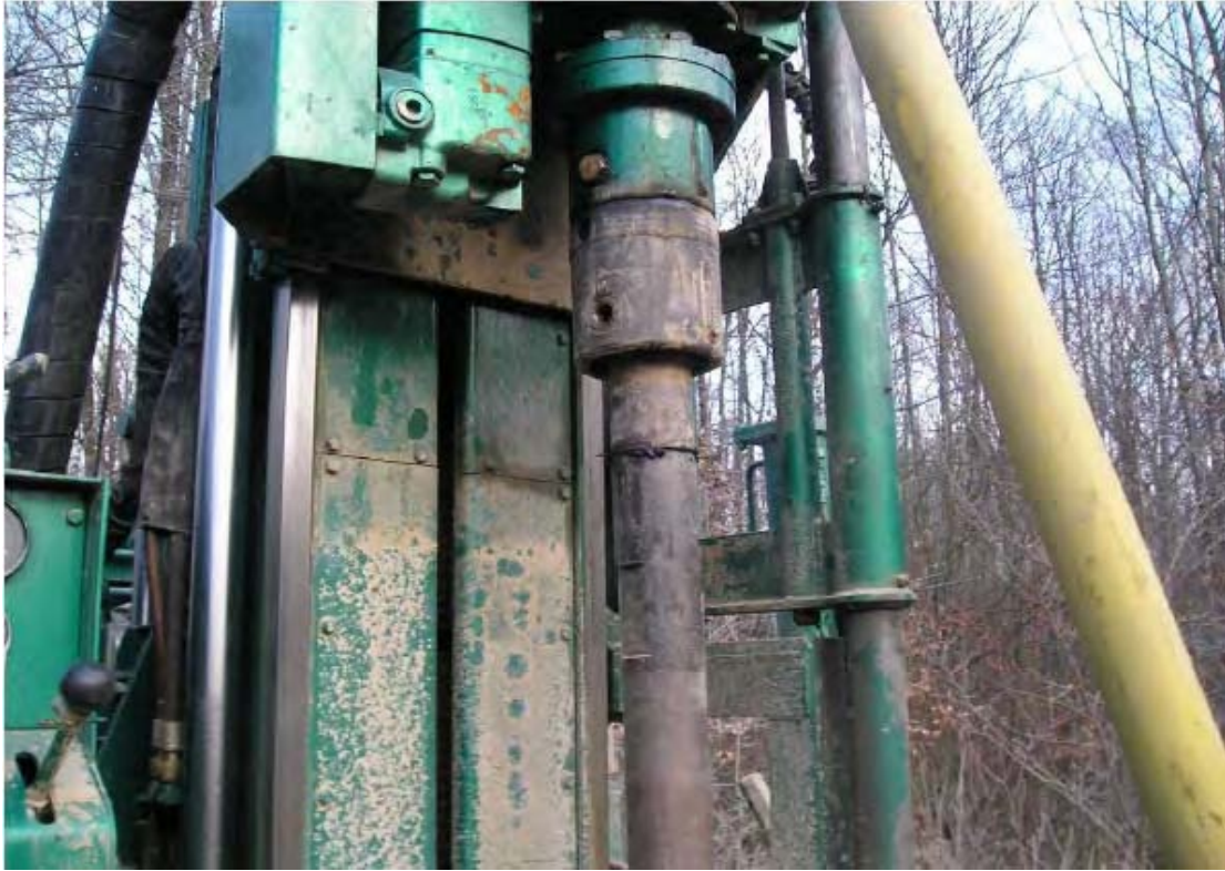
039 - Air rotary setup on the ATV rig.
