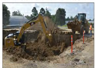
Some 1,500 cubic yards of soil were excavated, treated for contaminants and replaced during cleanup of a former motor pool site at the U.S. Army Engineer Research and Development Center in Vicksburg, Mississippi. The Vapor Energy Generator soil remediation system was used for the project, coordinated by the Omaha District. Photo by Kerry Larsen.
