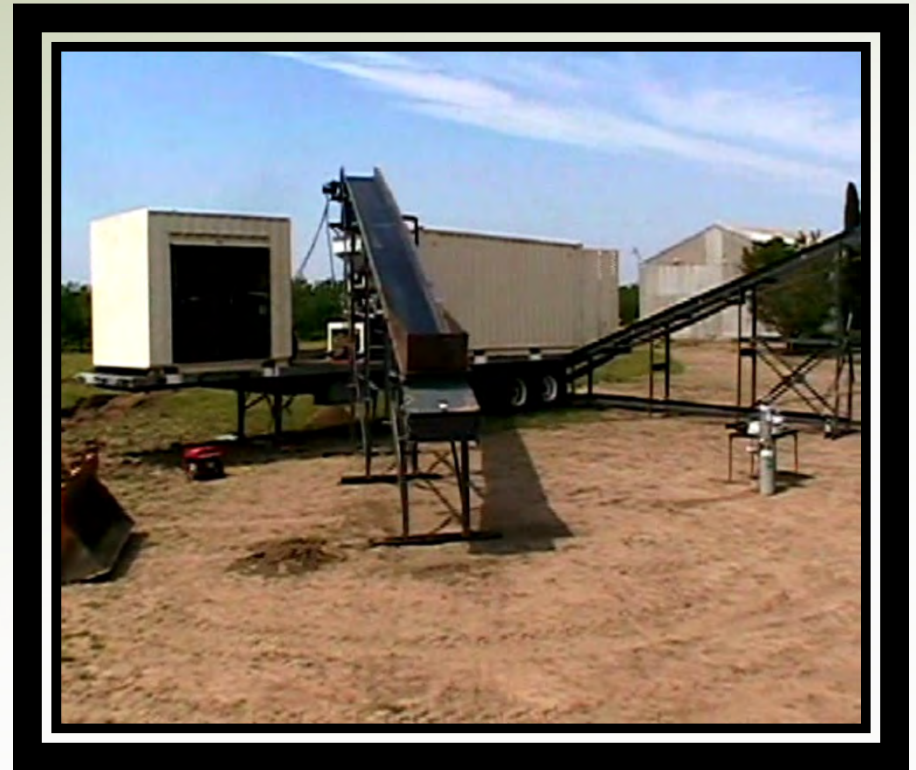
VEG Ex-Situ Soil Remediation System
