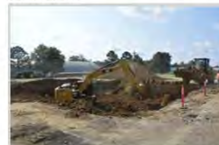
Twenty-five hundred cubic yards of soil were excavated, treated for contaminants and replaced during recent cleanup efforts on the former motor pool site at the U.S. Army Engineer Research and Development Center in Vicksburg, Miss. The Vapor Energy Generator soil remediation system was used for the project, coordinated by the U.S. Army Corps of Engineers Omaha District. (Photo by U.S. Army Corps of Engineers)
